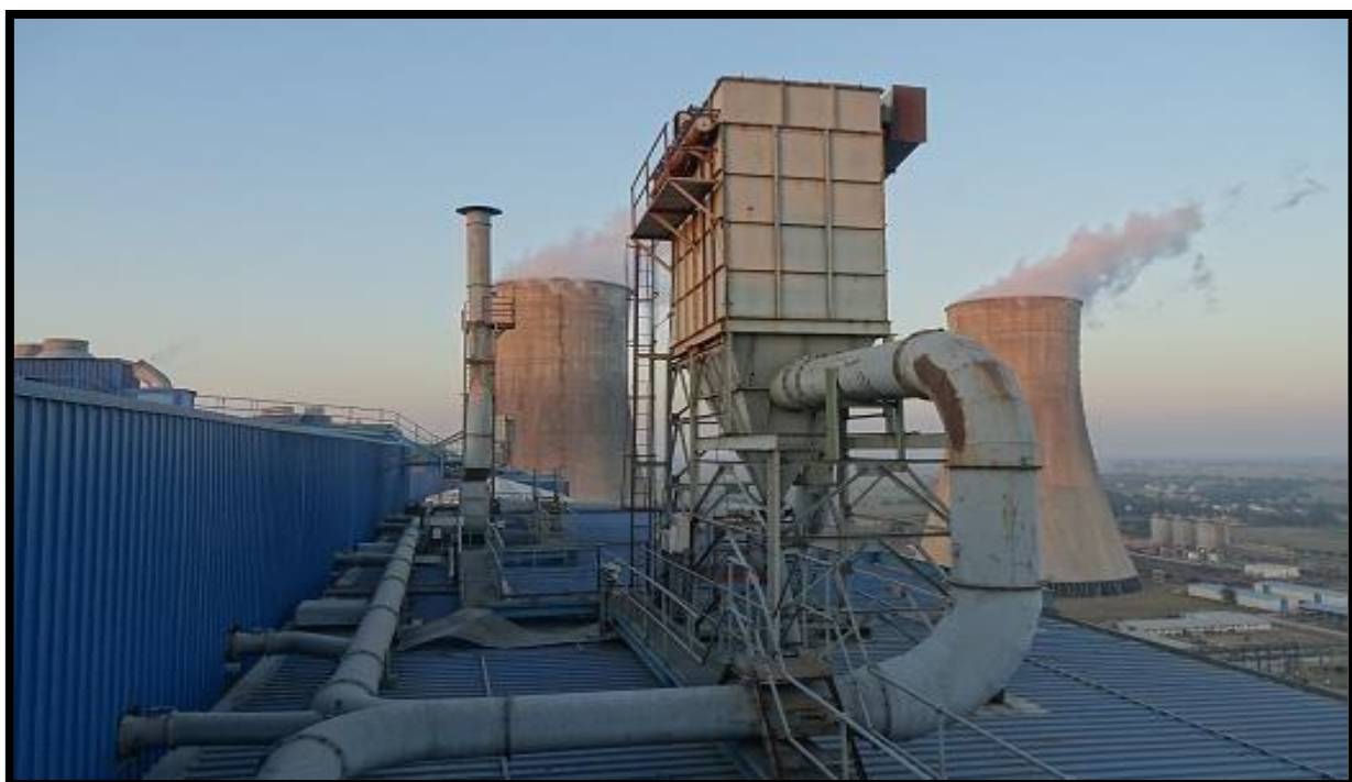
Dust Extraction System at Bunker
