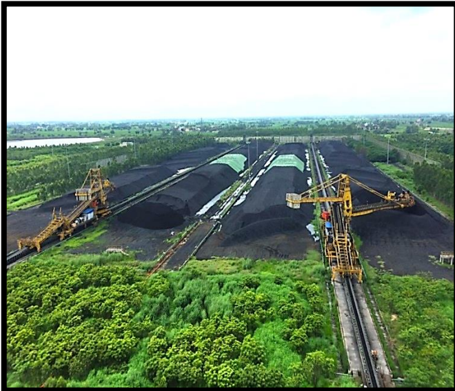
Pic-3 Three side coverage by wind screen to control fugitive emissions due to wind flow.
