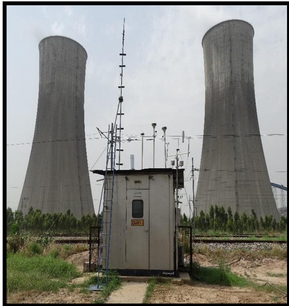
Pic-1 Four numbers of Continuous Ambient Air Quality Monitoring stations have been installed inside plant in consultation with PPCB officials to monitor ambient air quality.
