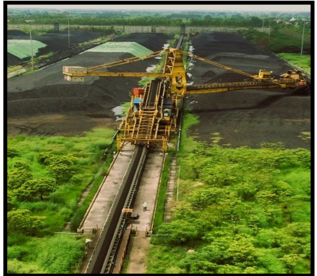
Pic-4 Automated and Mechanized Coal Handling System to minimize manual operations.
