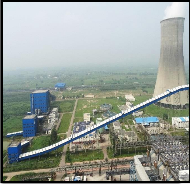
Pic-1 Covered conveyors for transfer of coal from Wagon tippler to coal bunkers for abatement of fugitive emissions.
