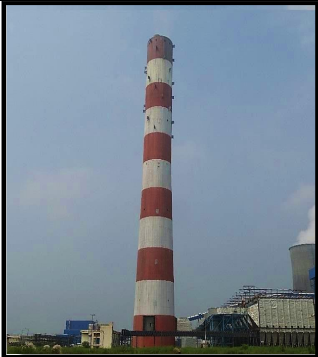
Pic-2. 275-meter-high Boiler stack for wider dispersion of dust and gaseous emissions
