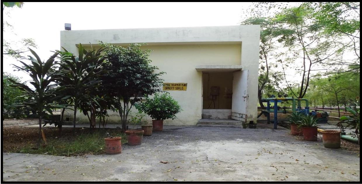
Pic-1 Sewage Treatment Plant
