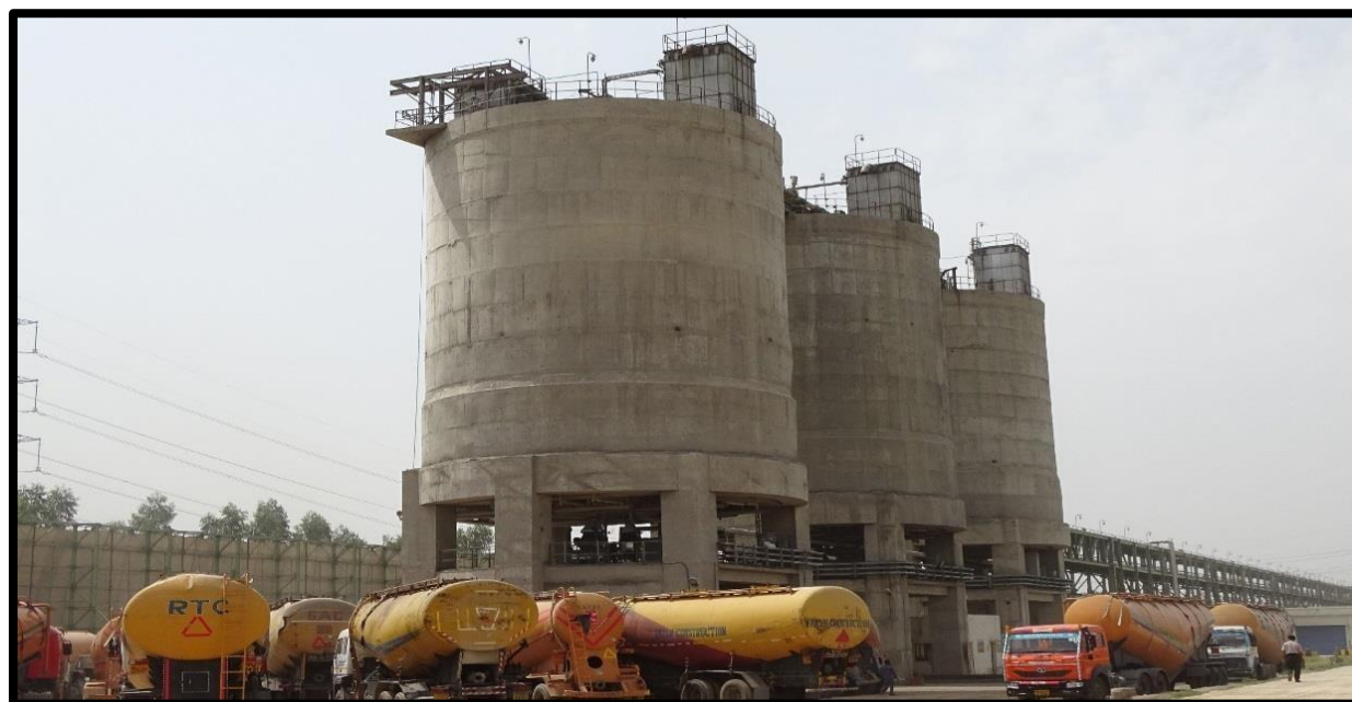
Pic-1 Transportation of Fly-ash in closed bulkers.
