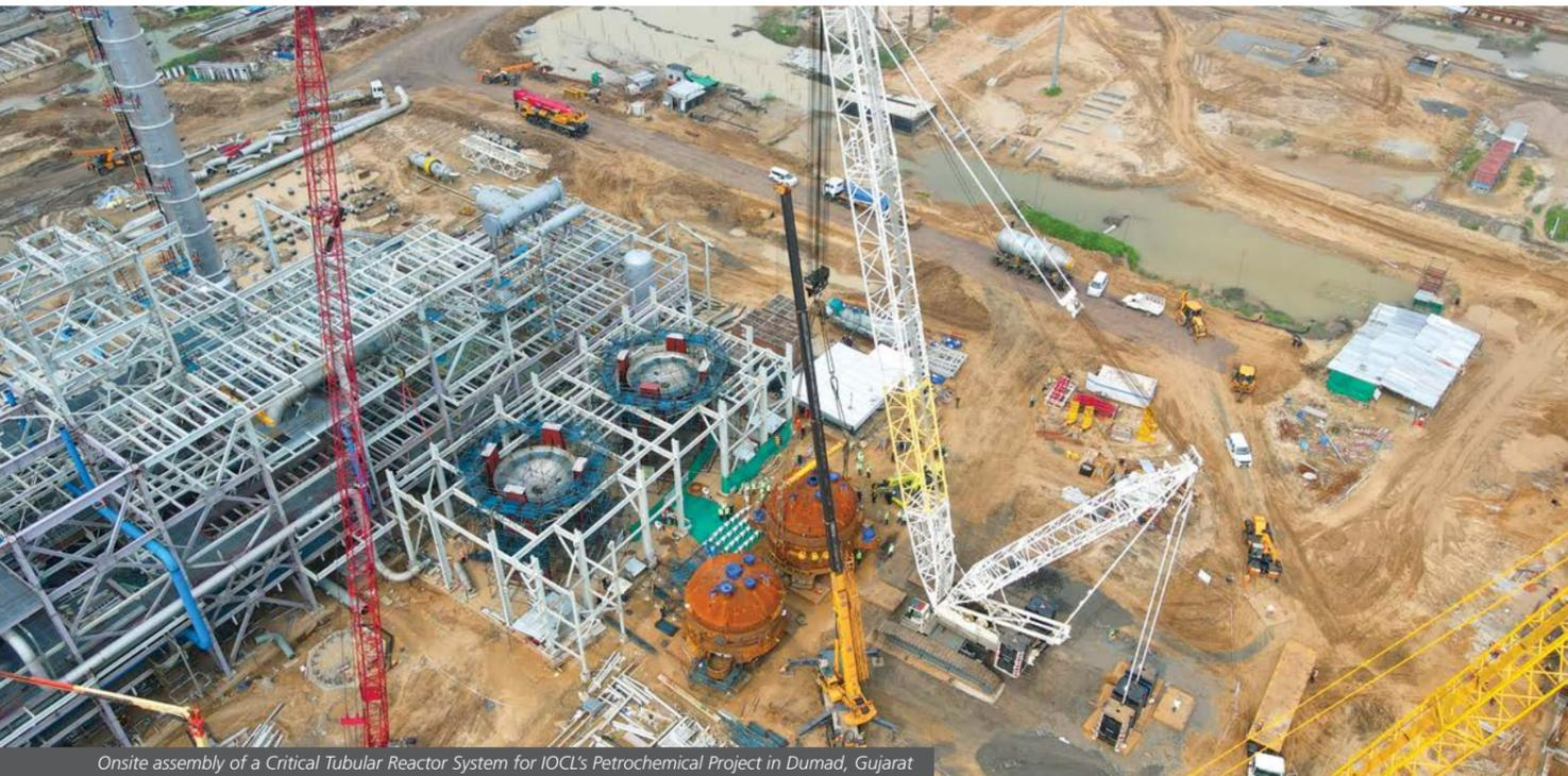
Onsite assembly of a Critical Tubular Reactor System for IOCL's Petrochemical Project in Dumad, Gujarat
