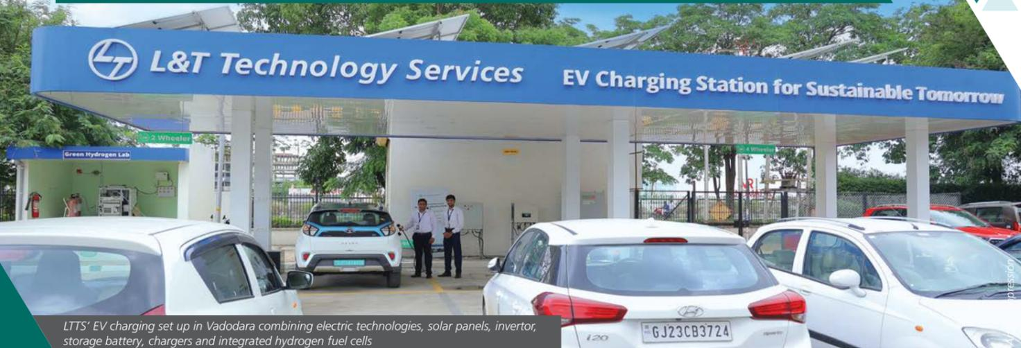
LTTS' EV charging set up in Vadodra combining electric technologies, solar panels, inverter, storage battery, chargers and integrated hydrogen fuel cells
