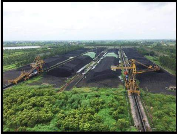
Pic-1 Green belt around coal stockpile area
