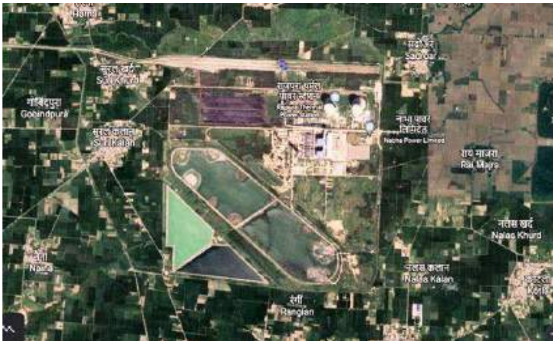
Figure 4: Google Image of Rajpura Power Project
