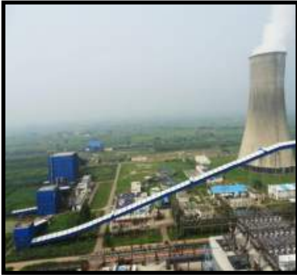
Covered conveyors for transfer of coal from Wagon tippler to coal bunkers for abatement of fugitive emissions
