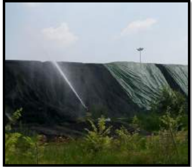
Dust suppression (sprinkler system) provided at each coal stockpile to arrest Dust
