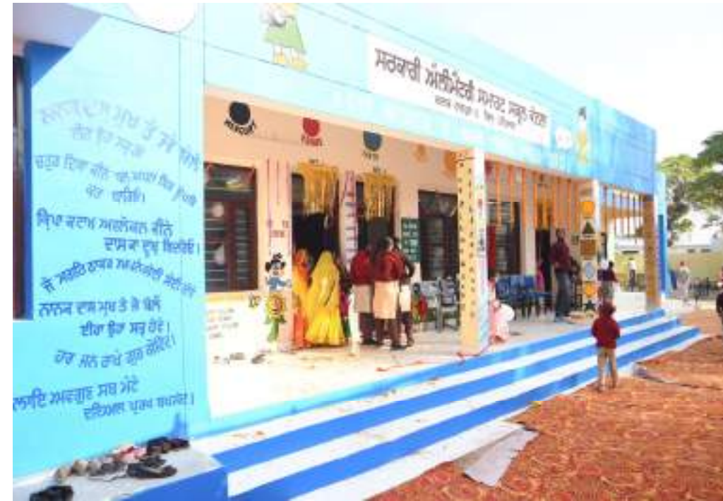
Construction of School Block in GES Kotla
