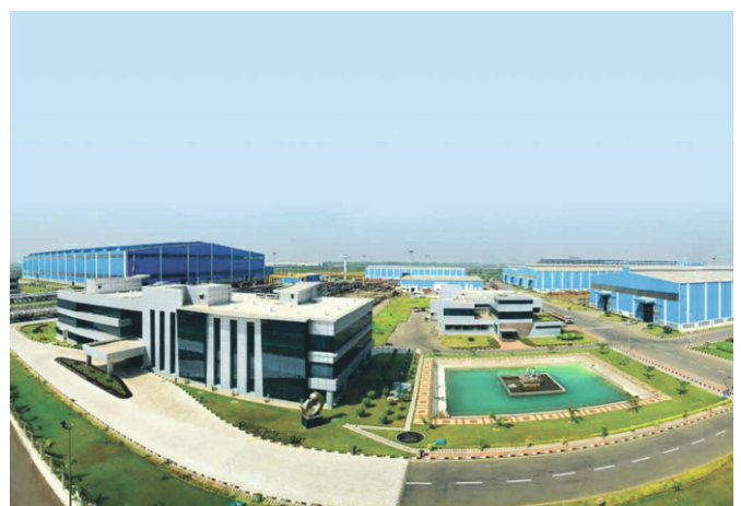
Power equipment making facility at A. M. Naik Heavy Engineering Complex, Hazira
