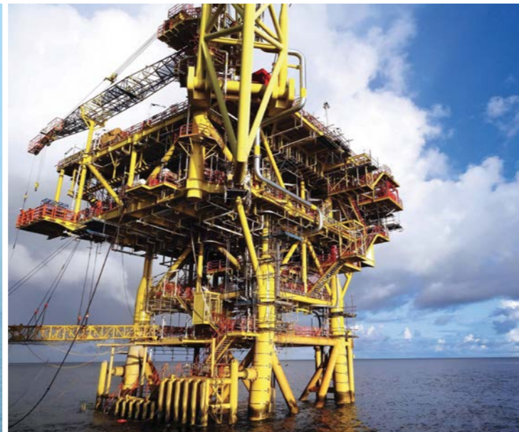
Yetagun 'D' Platform installed offshore for PETRONAS Carigali
