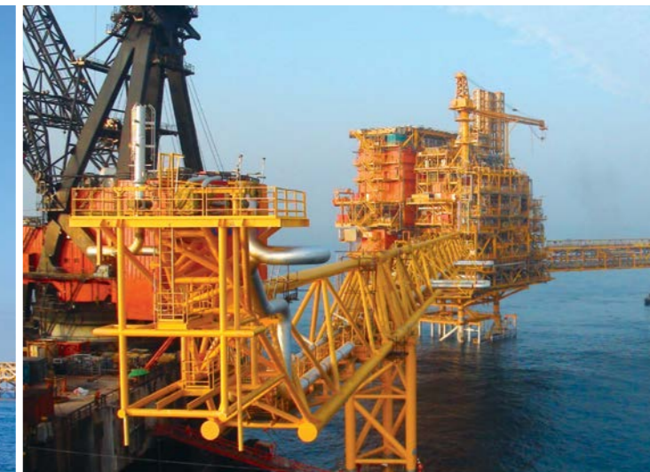
DDW1 Wellhead Platform & Process-cum-living Quarters Platform for GSPC, installed off India's east coast
