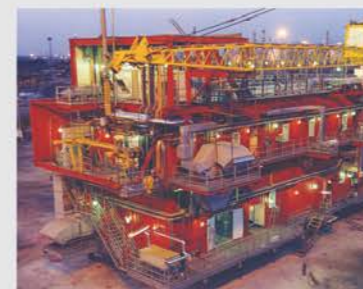
Living Quarter Modules & E-Houses
