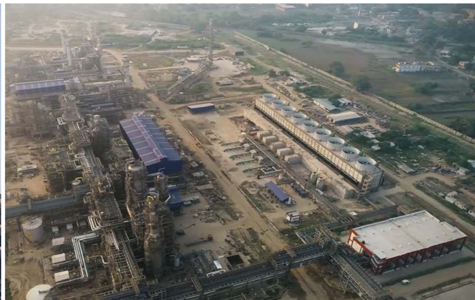
Intigrated Ammonia-Urea Complex for Hindustan Urvarak Rasayan Limited, Barauni, India
