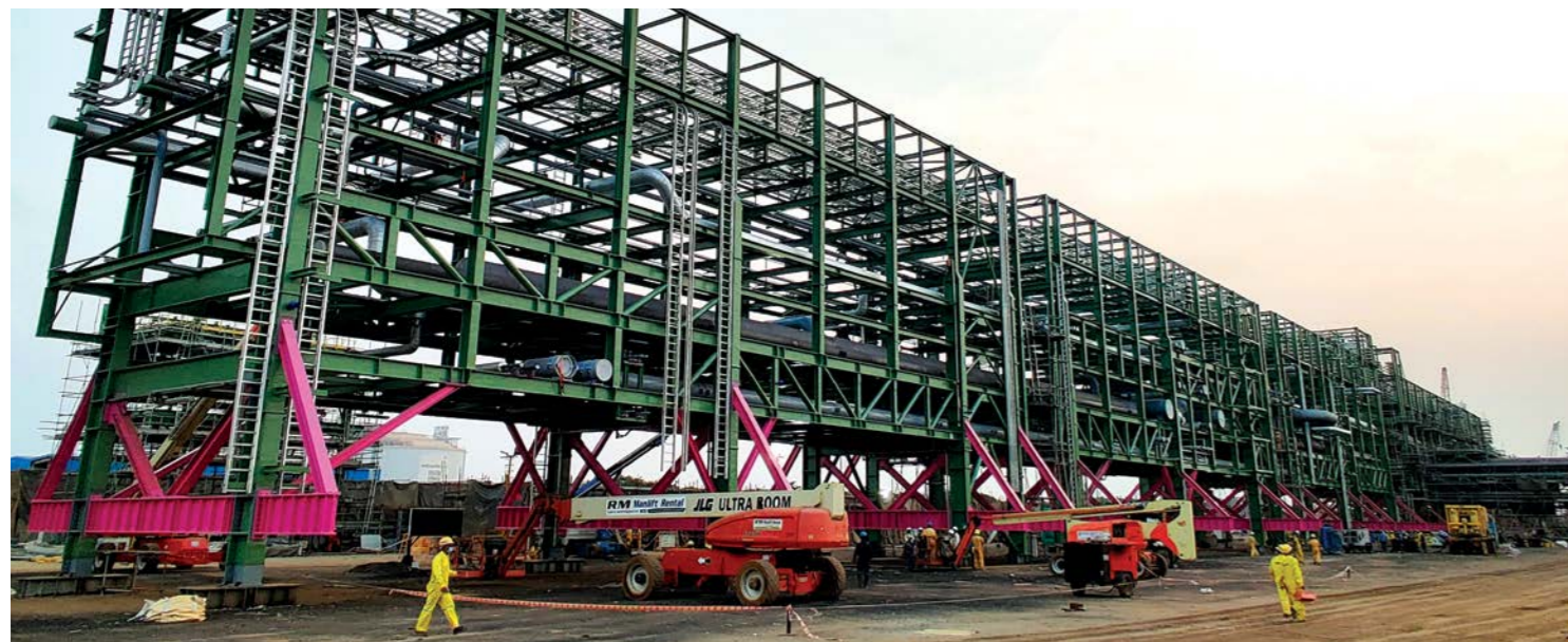
Onshore Process and Pipe Rack Modules being readied at MFF-Kattupalli
