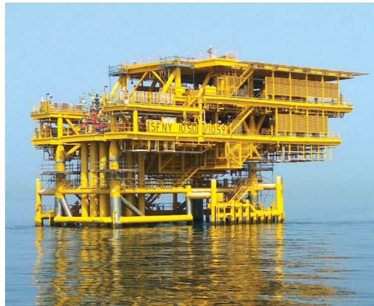
One of the 4 Decks of SFNY-4D project installed in Safania Field for Saudi Aramco
