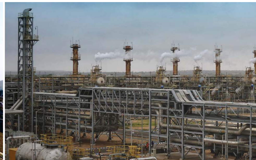
Cairn Mangala Upgradation Facility – II project, Barmer
