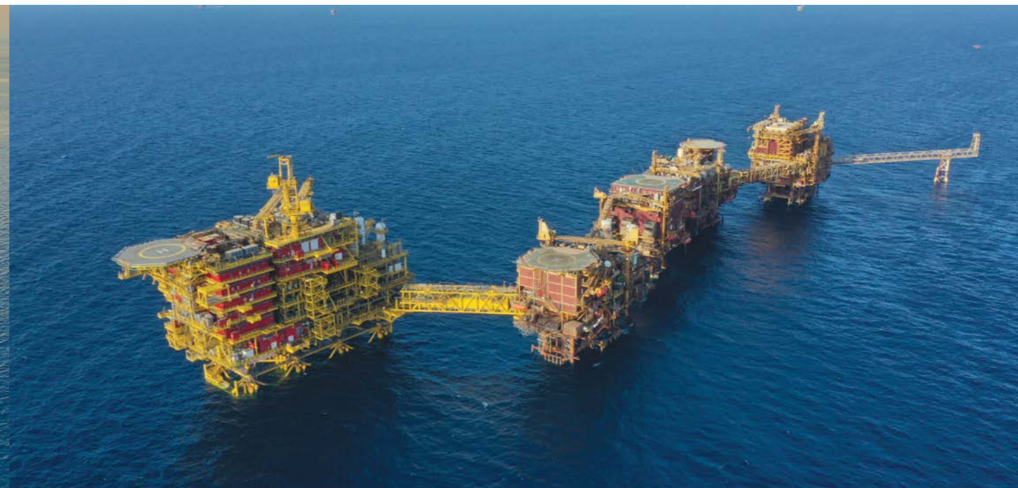
New Water Injection South (NWIS - R) Project for ONGC
