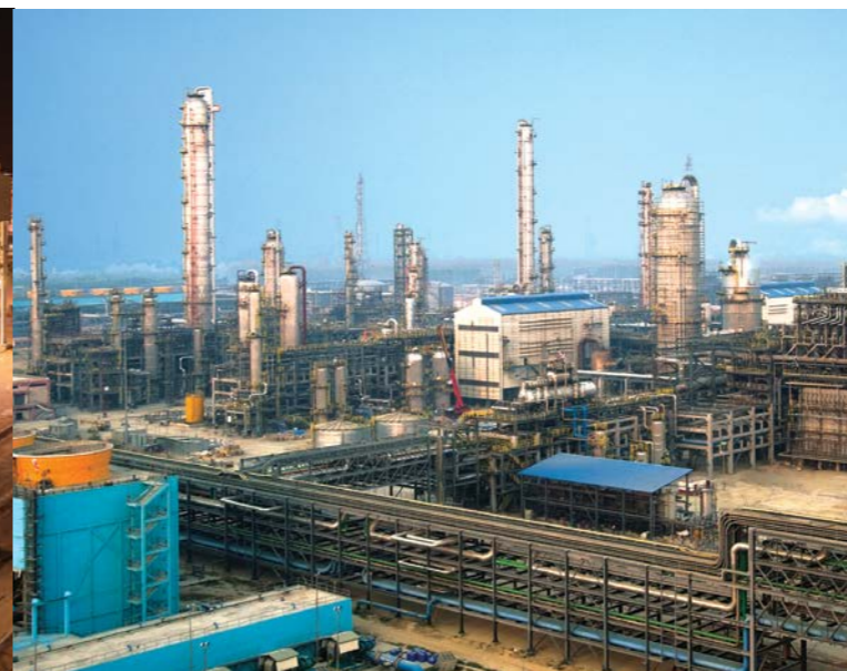
Naphtha Cracker & Associated Units for IOCL's Panipat Refinery, India
