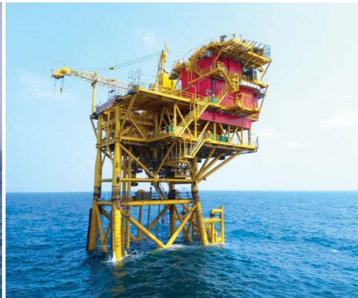
One of the 3 wellhead platforms of Bassein Development 3 Project for ONGC
