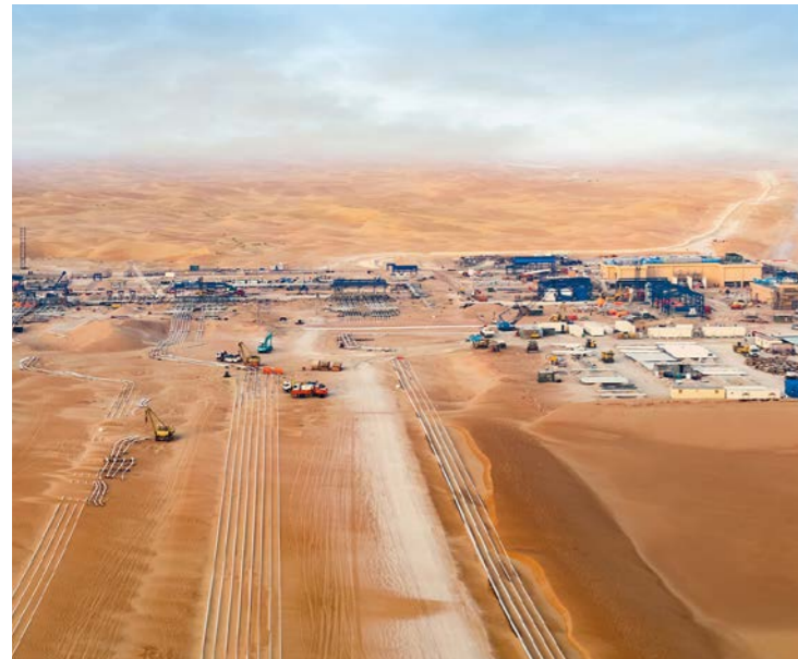
Haliba Field Development Project for Al-Dhafa Petroleum Operations, Abu Dhabi, UAE
