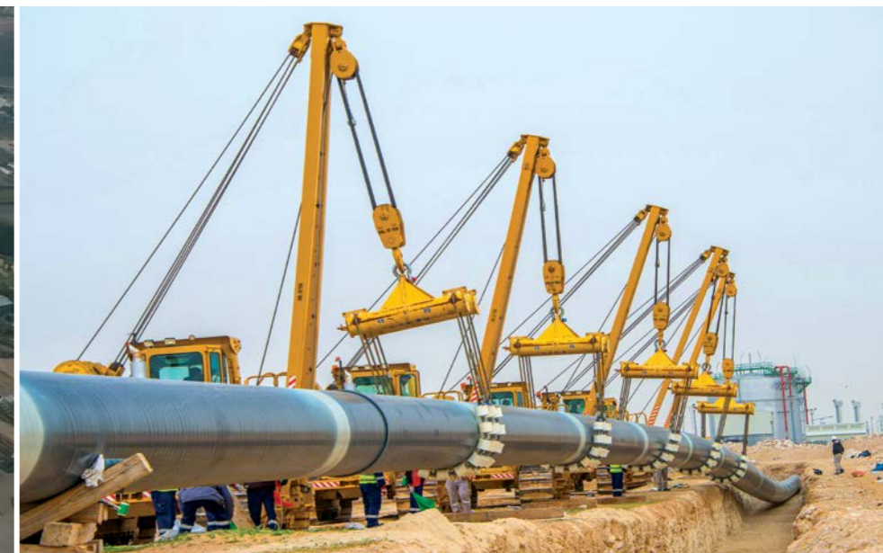
48" x 118 km-long Crude Transit Line from North Kuwait to Central Mixing Manifold for KOC, on EPC basis
