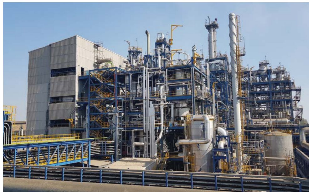
40,000 MTPA Melamine Plant for Gujarat State Fertilizers & Chemicals, Vadodara, India
