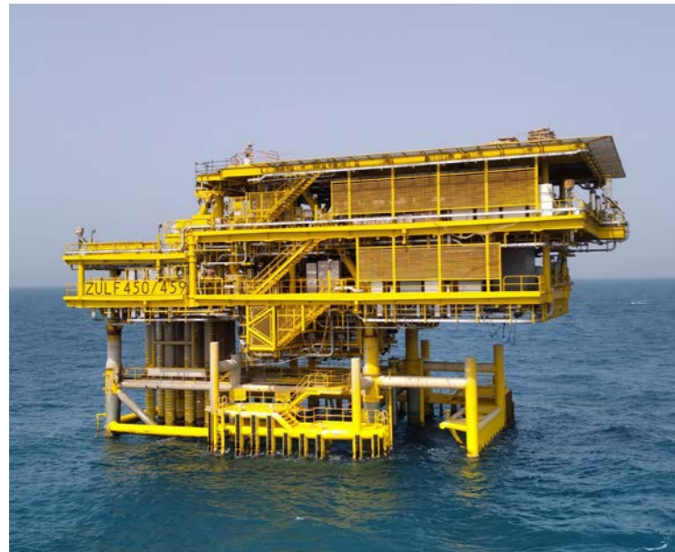
Two Oil PDMs and Associated Facilities in Zuluf Field for Saudi Aramco
