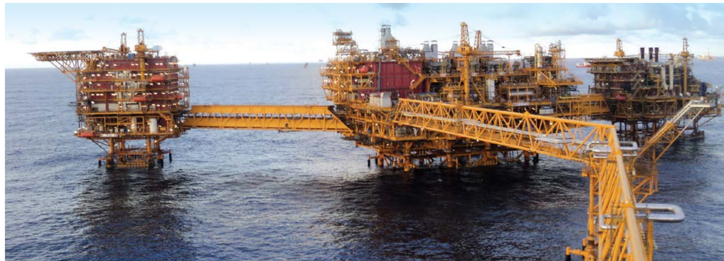
Mumbai High North Complex of ONGC, executed by L&T on an EPCIC basis. The massive complex comprises a 26,500 MT process platform, a living quarters platform and control room, three process gas compression platforms, two flare platforms and two jackets – including one weighing 13,500 tonnes
