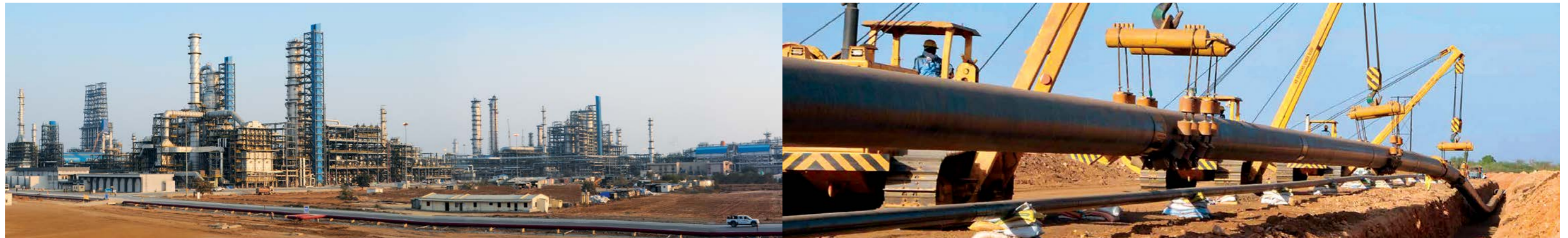
Panoramic view of HREL Bhatinda Refinery, India. Scope included EPC of 2 x 44,000 MTPA Hydrogen Generation Units and mechanical construction of 7 processing units
