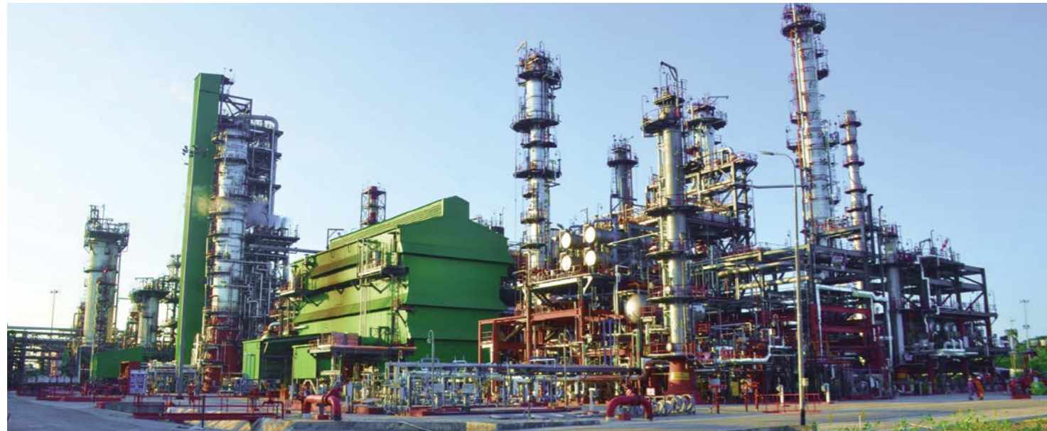
INDMAX FCC Unit including LPG Treatment Facility for IOCL at Bongaigaon, India.
