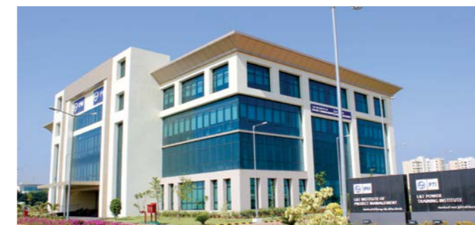
L&T Institute of Project Management (IPM) at Vadodara – a registered educational provider of PMI, USA – develops project managers across EPC domains
