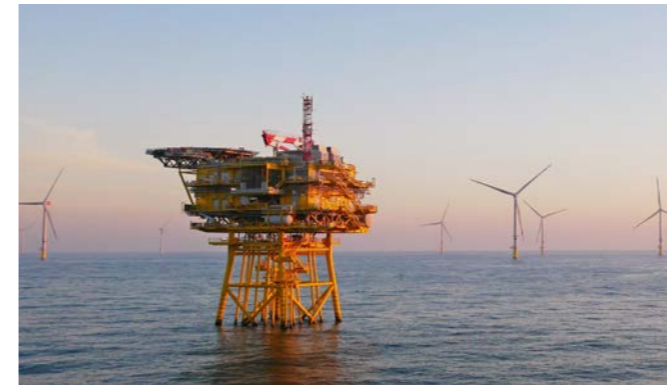
Offshore Substation Platform
