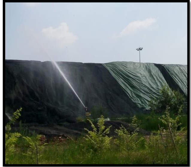
Dust suppression (sprinkler system) provided at each coal stockpile to arrest Dust
