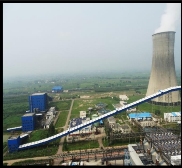
Covered conveyors for transfer of coal from Wagon tippler to coal bunkers for abatement of fugitive emissions
