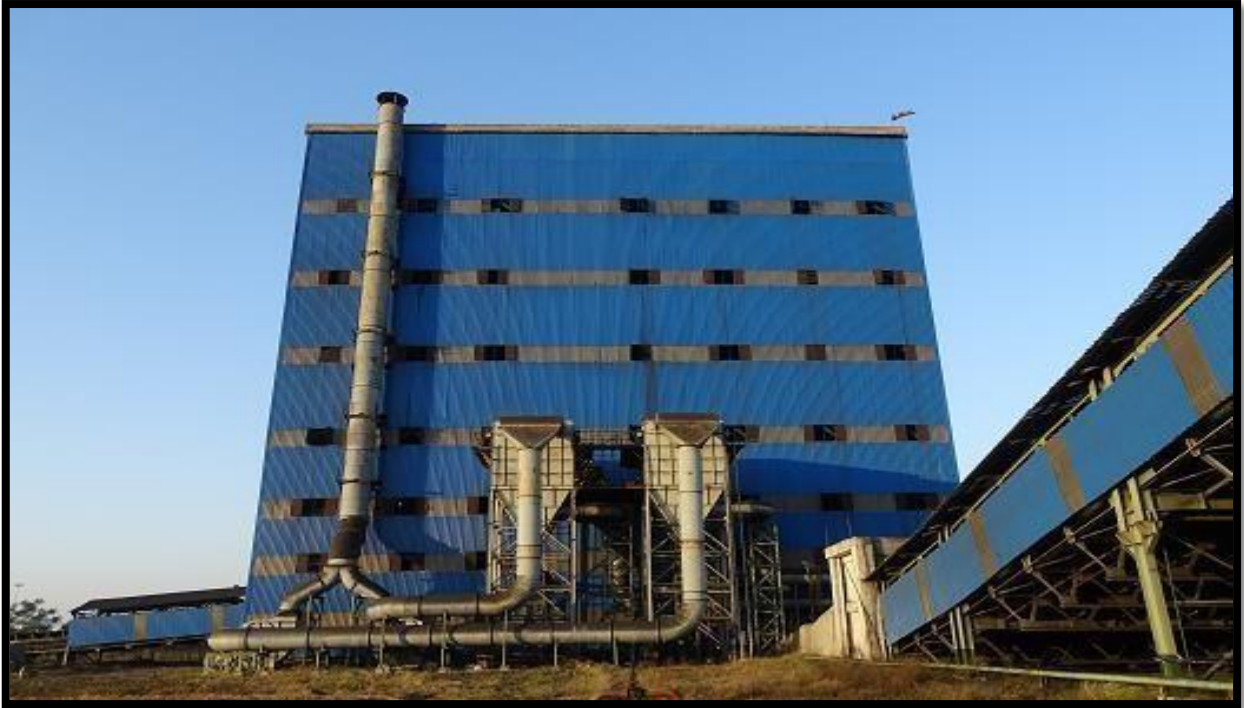
Dust Extraction System at Crusher House
