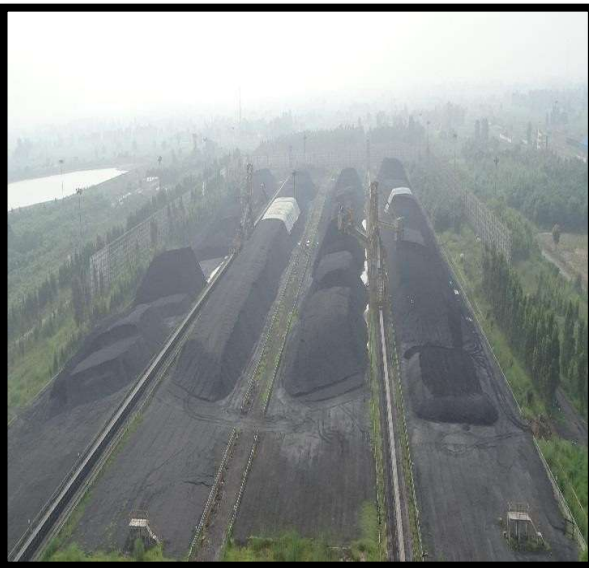
Pic-3 Three side coverage by wind screen to control fugitive emissions due to wind flow.
