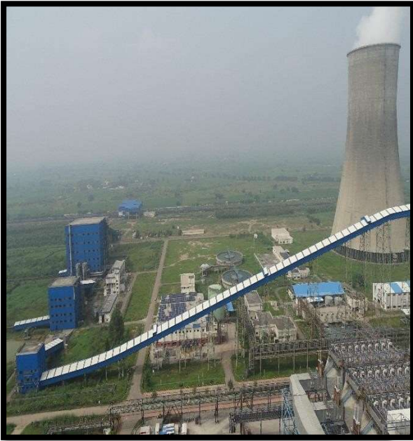
Pic-1 Covered conveyors for transfer of coal from Wagon tippler to coal bunkers for abatement of fugitive emissions.
