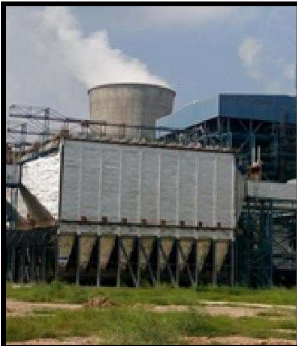
Pic-1. High efficiency ESP (99.99%) to control particulate matter
