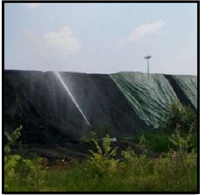
Pic-2 Dust suppression (sprinkler system) provided at each coal stockpile to arrest Dust.
