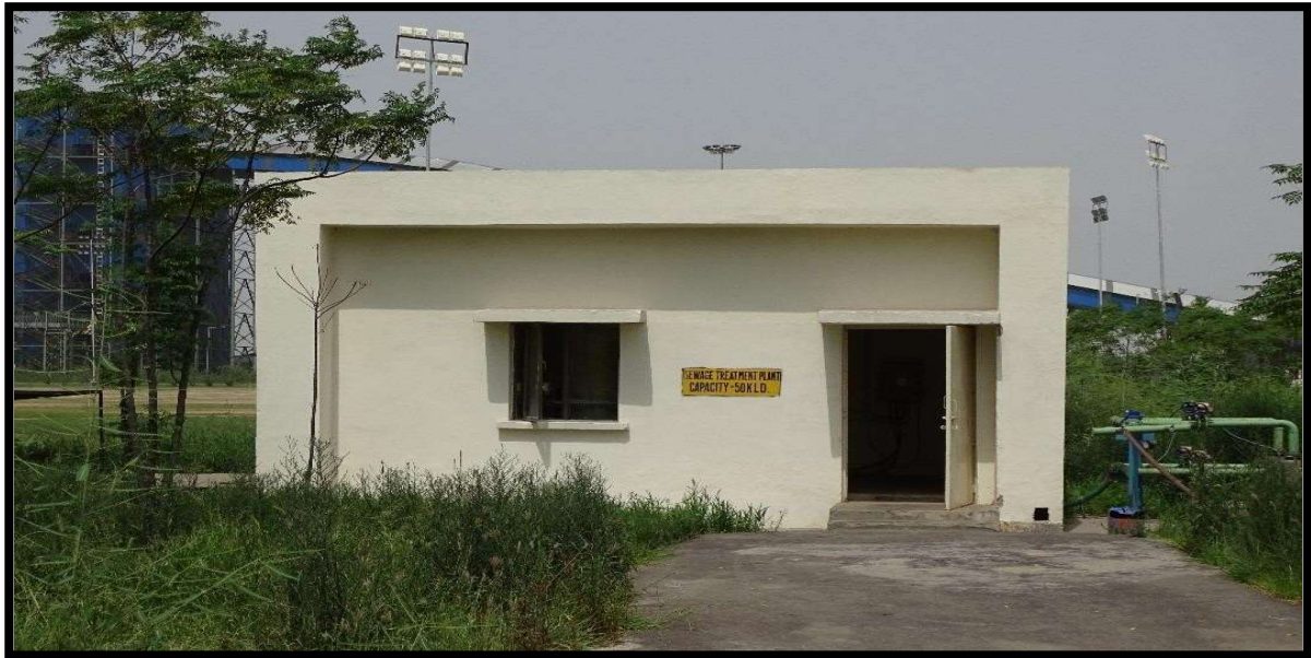
Pic-1 Sewage Treatment Plant
