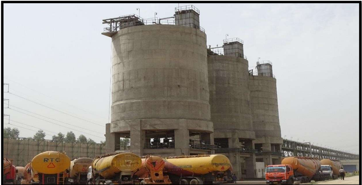
Pic-1 Transportation of Fly-ash in closed bulkers.
