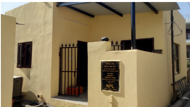
EWS House built at Village Bhappal
