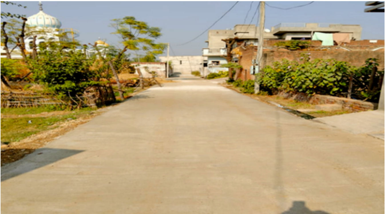
Road Development project at Village Bakshiwala
