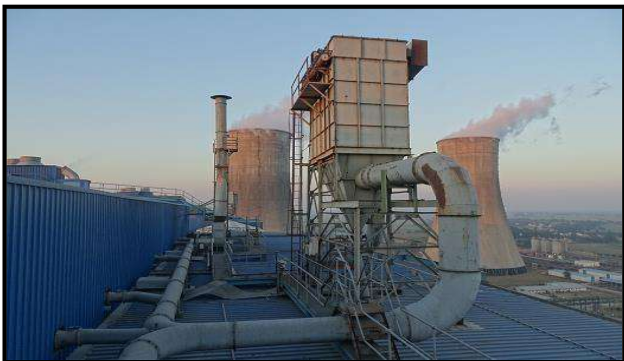
Dust Extraction System at Bunker
