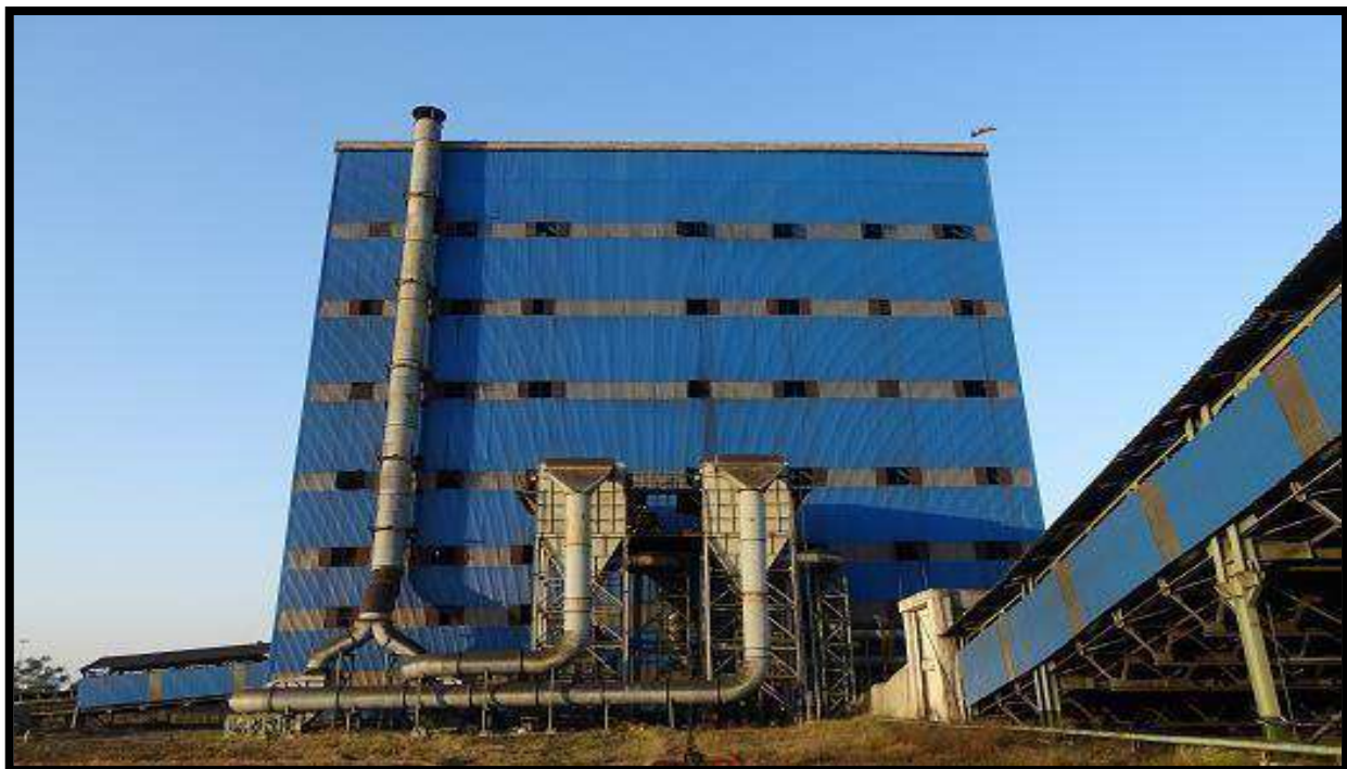
Dust Extraction System at Crusher House
