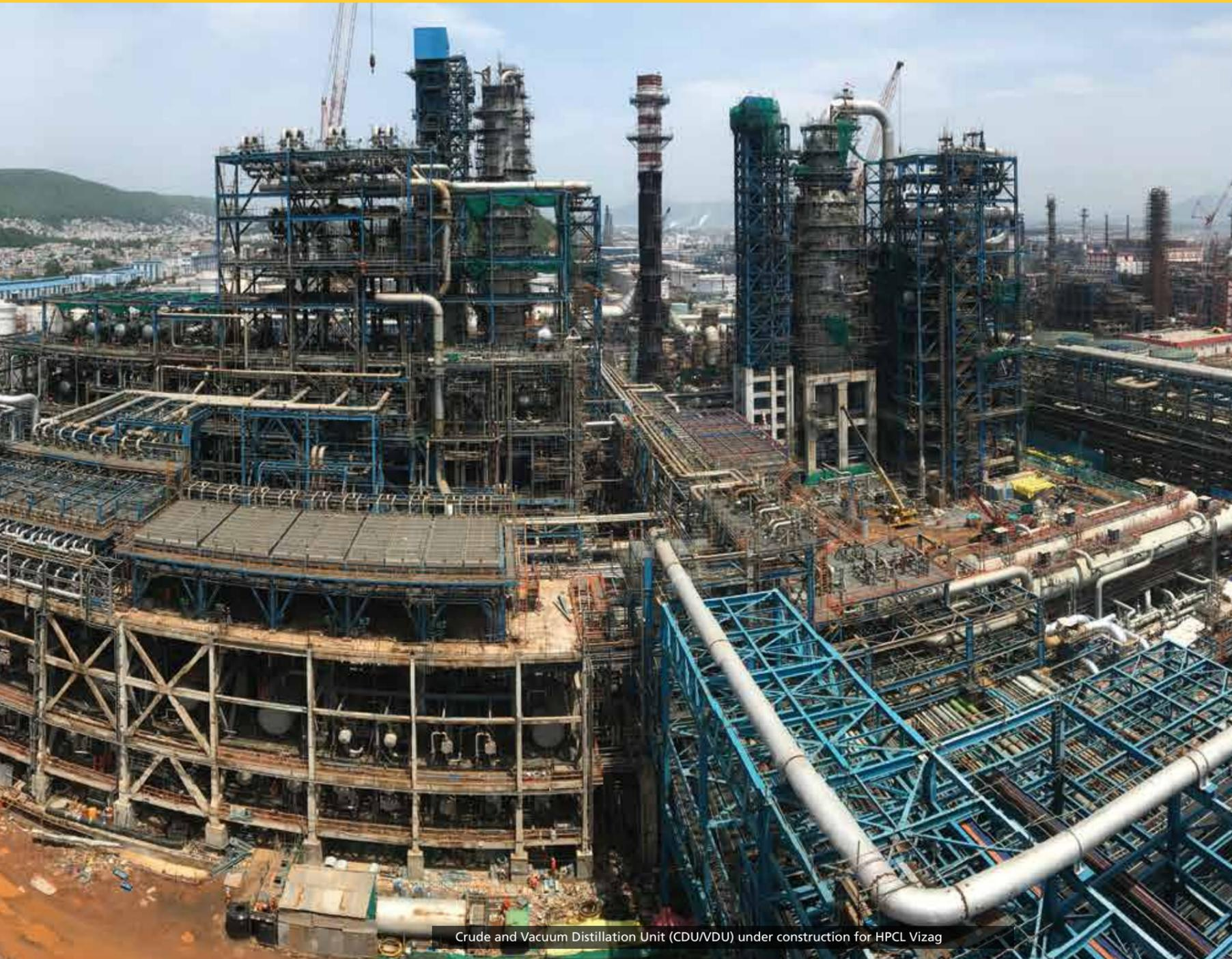
Crude and Vacuum Distillation Unit (CDU/VDU) under construction for HPCL Vizag
