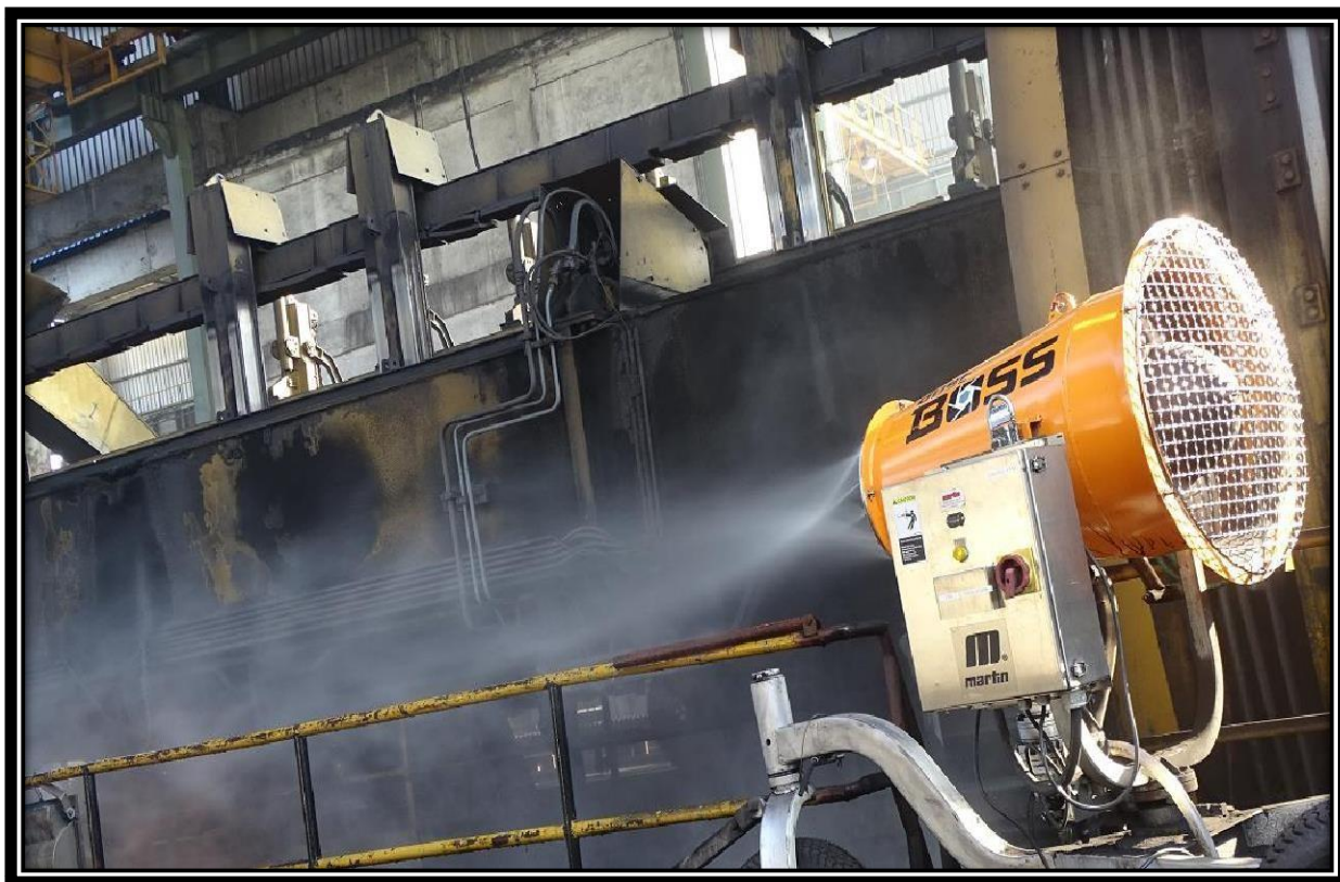
Dust Suppression System installed at Wagon Tippler Area to control Fugitive Emission During Unloading of Coal.
