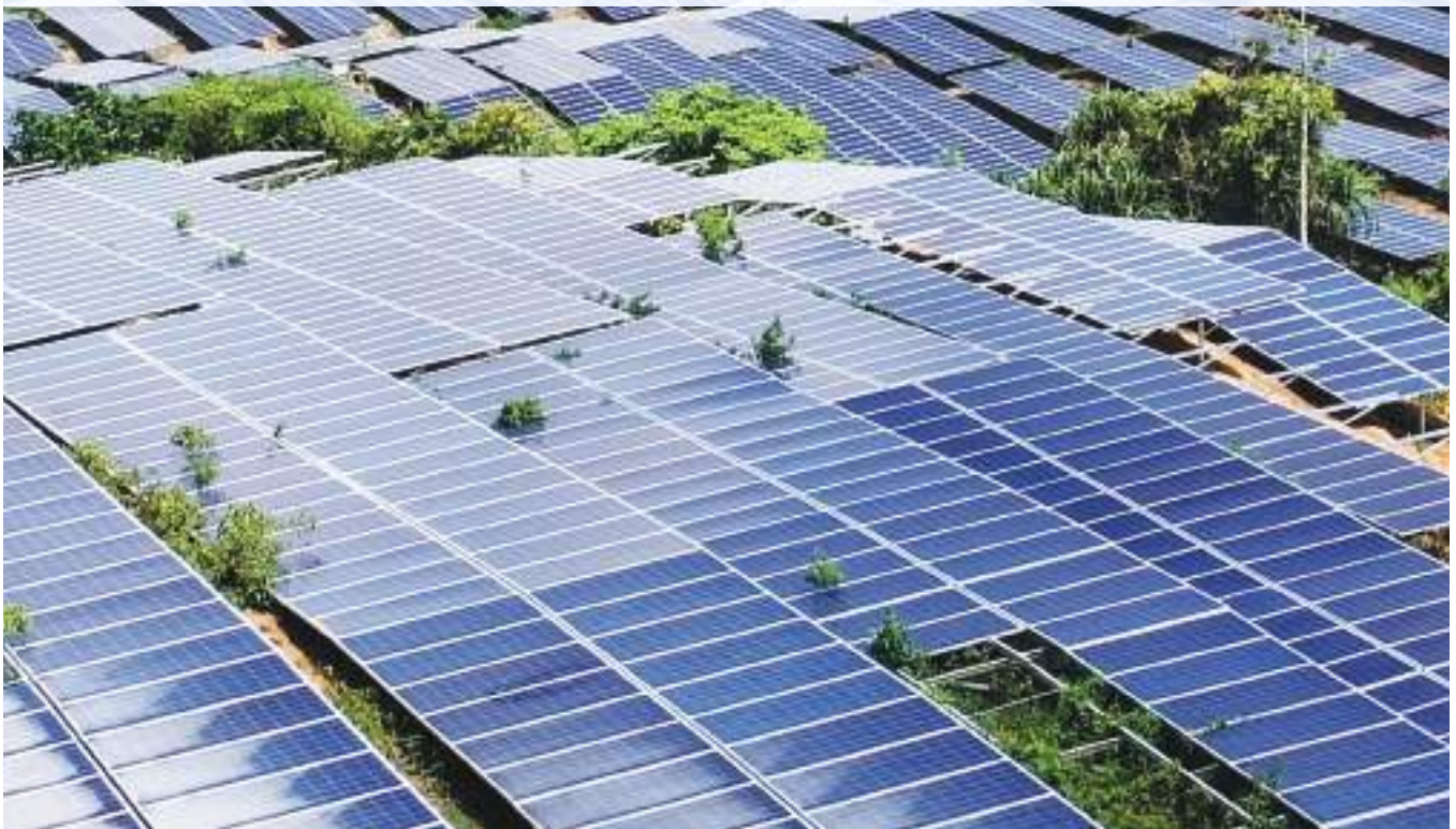
India's first large-scale solar PV project of 2 x 10 MW with 16 MW/8 MWh battery energy storage system in the Andamans
