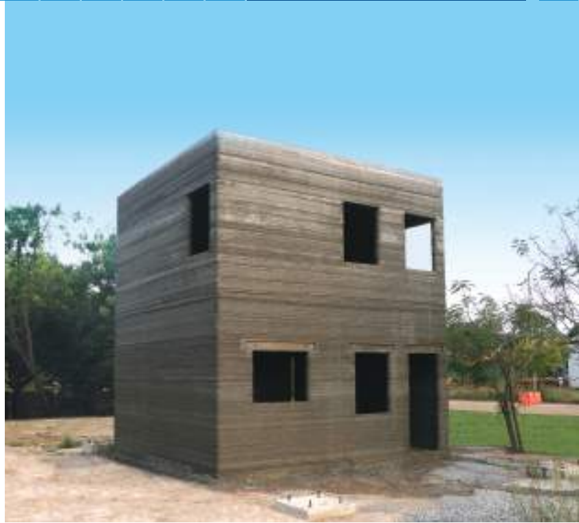
Use of 3D printing in construction
