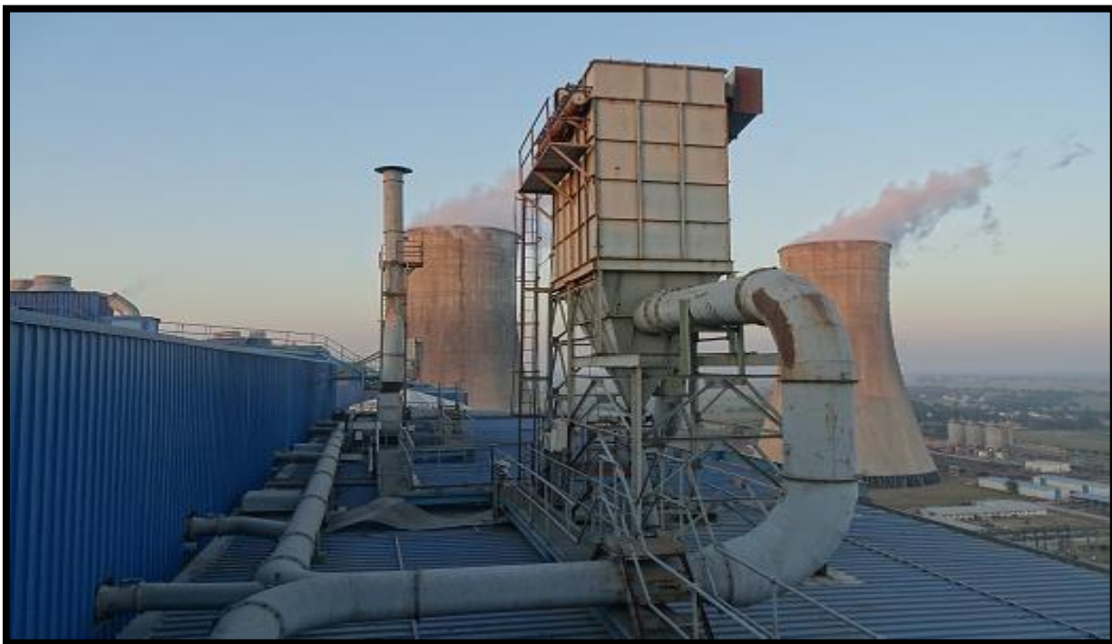
Dust Extraction System at Bunker
