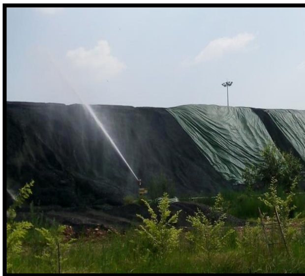
Dust suppression (sprinkler system) provided at each coal stockpile to arrest Dust
