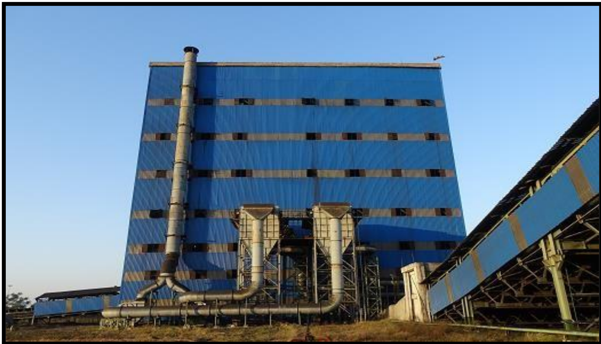
Dust Extraction System at Crusher House
