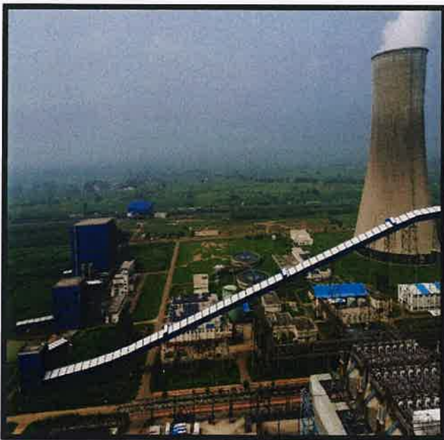
Pic-1 Covered conveyors for transfer of coal from Wagon tippler to coal bunkers for abatement of fugitive emissions
