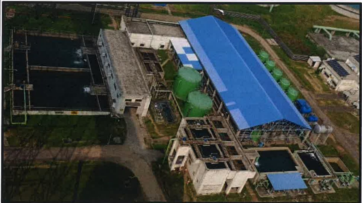
Pic-1 Effluent Treatment Plant
