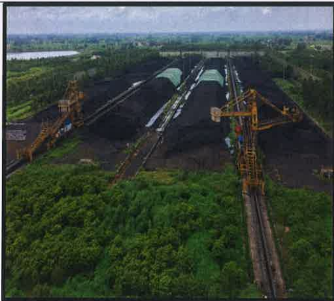
Pic-3 Three side coverage by wind screen to control fugitive emissions due to wind flow
