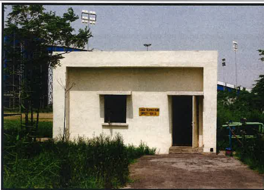
Pic-1 Sewage Treatment Plant
