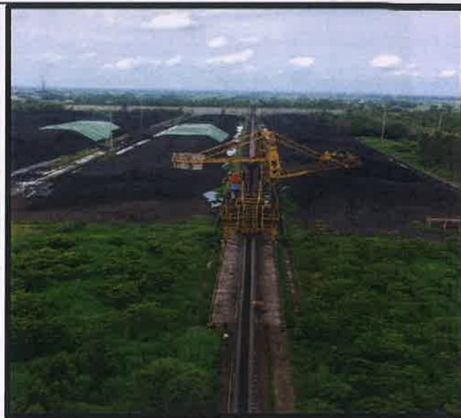
Pic-4 Automated and Mechanized Coal Handling System to minimize manual operations
