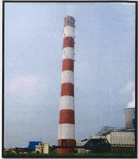
Pic-2 275-meter high Boiler stack for wider dispersion of dust and gaseous emissions
