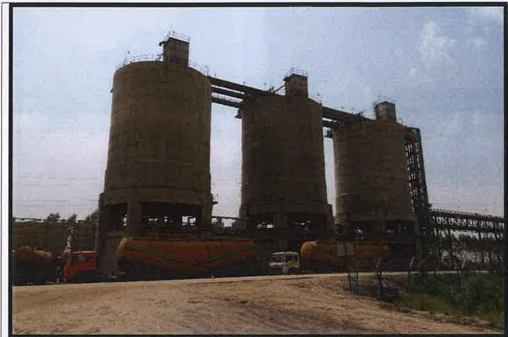
Pic-1 Transportation of Fly-ash in closed bulkers
