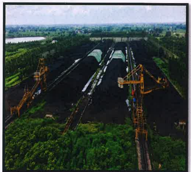
Three side covered windscreen to control fugitive emissions due to wind flow
