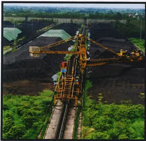
Automated and Mechanized Coal handling System to minimize manual operations
