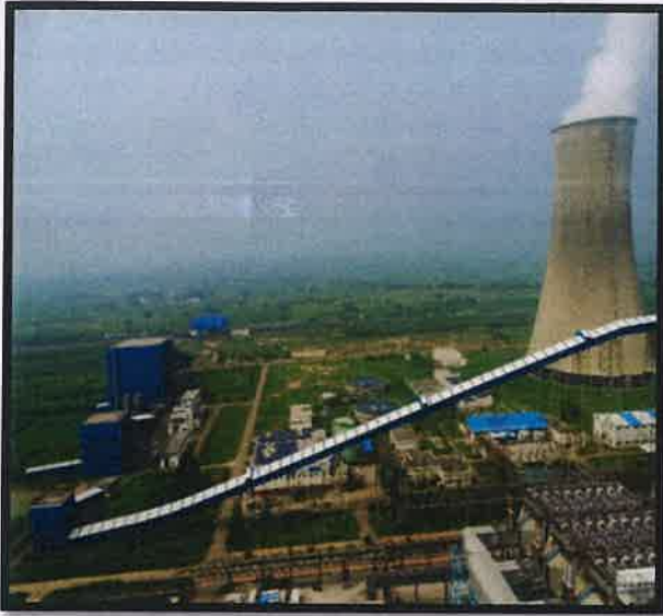
Covered conveyors for transfer of coal from Wagon tippler to coal bunkers for abatement of fugitive emissions
