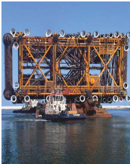
Sail-away of Asia's largest Process Platform jacket (13,500 MT) from the Oman yard
