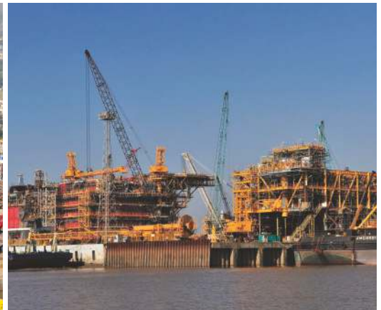
Fabrication of a process platform for ONGC's MHN Project at the yard
