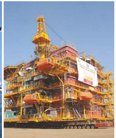
Load-out of India's heaviest offshore module (4300 MT) – 150-man Living Quarters for ONGC
