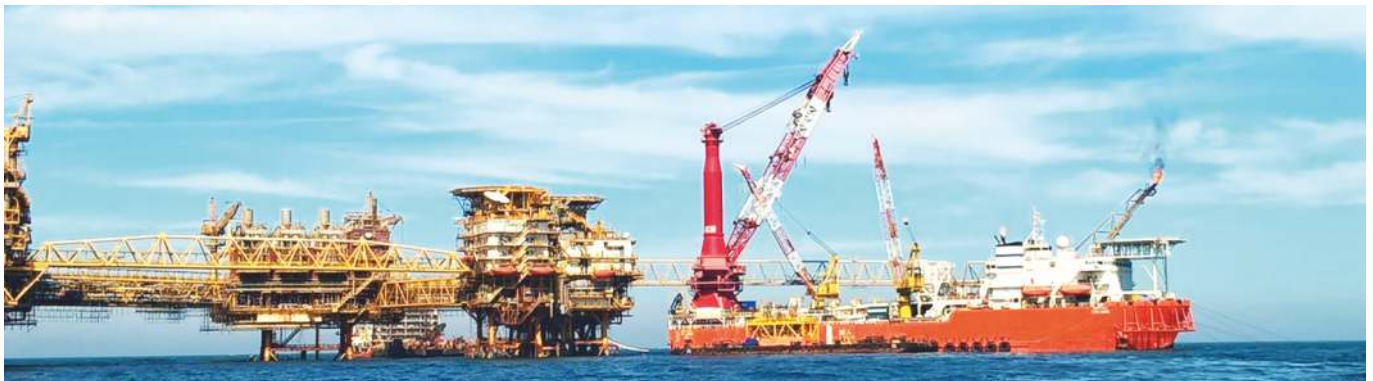
Additional Development of Vasai East Project on India's West Coast for ONGC. The scope included EPCIC of 2 Wellhead Platforms, 35 km Pipelines and modification. Picture also shows LTS 3000 – a captive heavy lift-cum-pipelay vessel.
