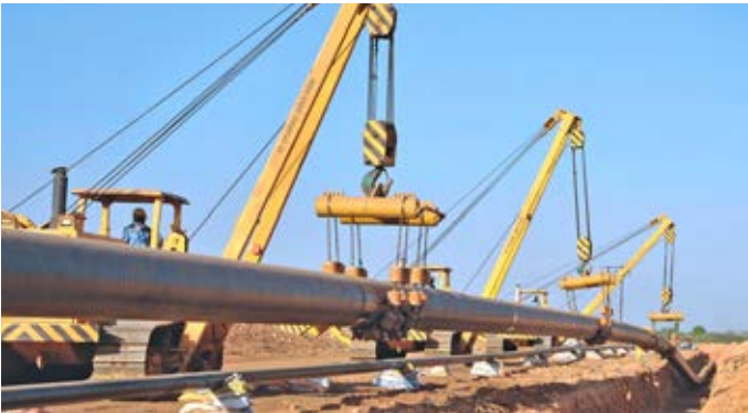
The world's longest heated and insulated waxy crude oil pipeline in India from Barmer to Bhogat (24" x 619 km crude oil pipeline and 8" x 527 km natural gas pipeline)
