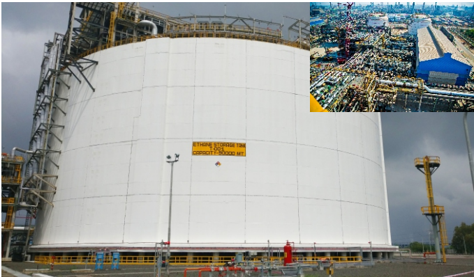
Ethane / LNG Dual Service Storage Tank for Reliance Industries, Dahej, India. Inset: Balance of Plant for Ethane Receipt & Storage
