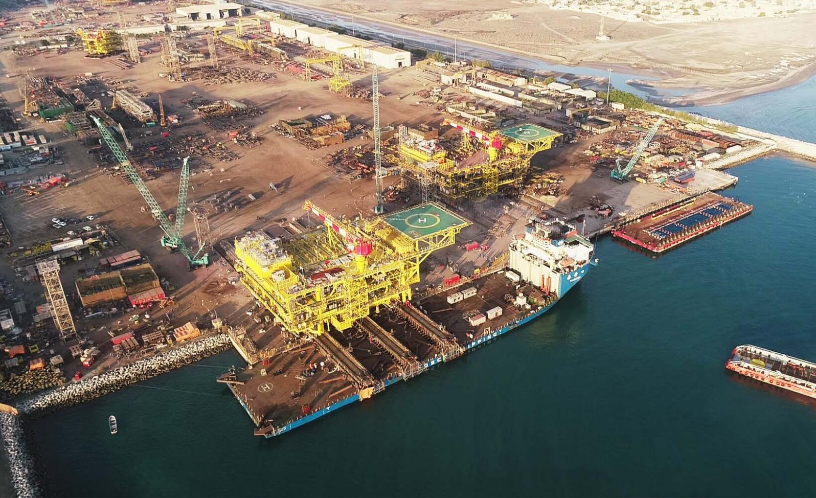
*Load-out of two mega Tie-in Platforms (7000 MT each) for Hasbah Field, Saudi Aramco from L&T Hydrocarbon Engineering's Oman facility*
