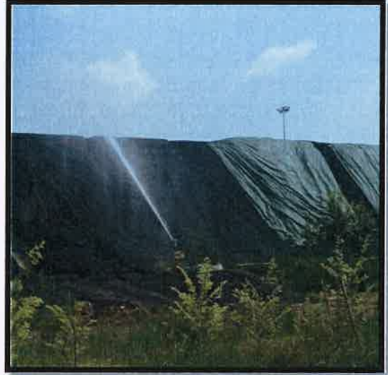
Dust suppression (sprinkler system) provided at each coal stockpile to arrest Dust
