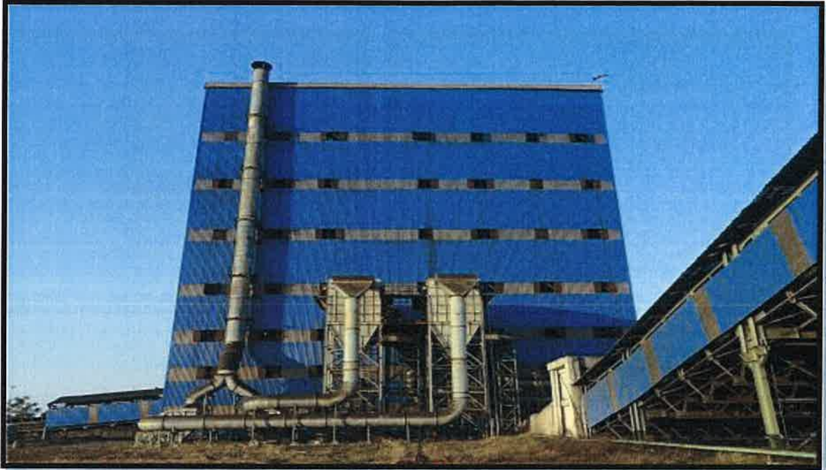
Dust Extraction System at Crusher House
