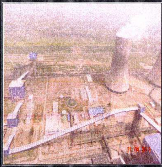
Covered conveyors for transfer of coal from Wagon tippler to coal bunkers for abatement of fugitive emissions
