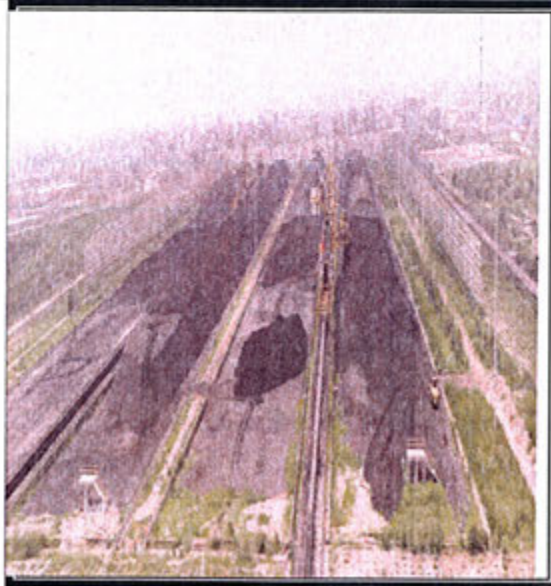
Three side covered wind screen to control fugitive emissions due to wind flow
