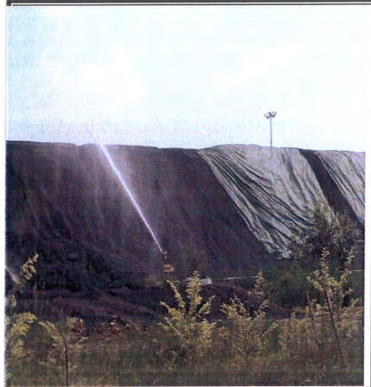
Dust suppression (sprinkler system) provided at each coal stock pile to arrest Dust
