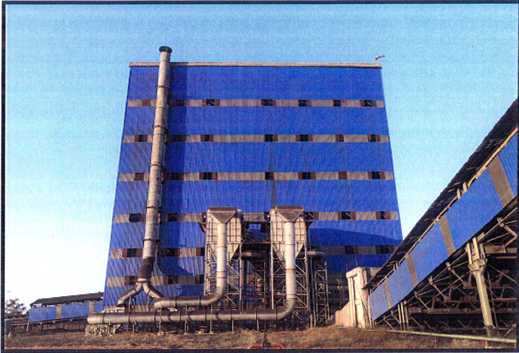
Dust Extraction System at Crusher House
