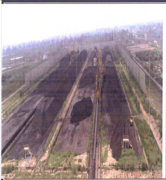
Three side covered wind screen to control fugitive emissions due to wind flow
