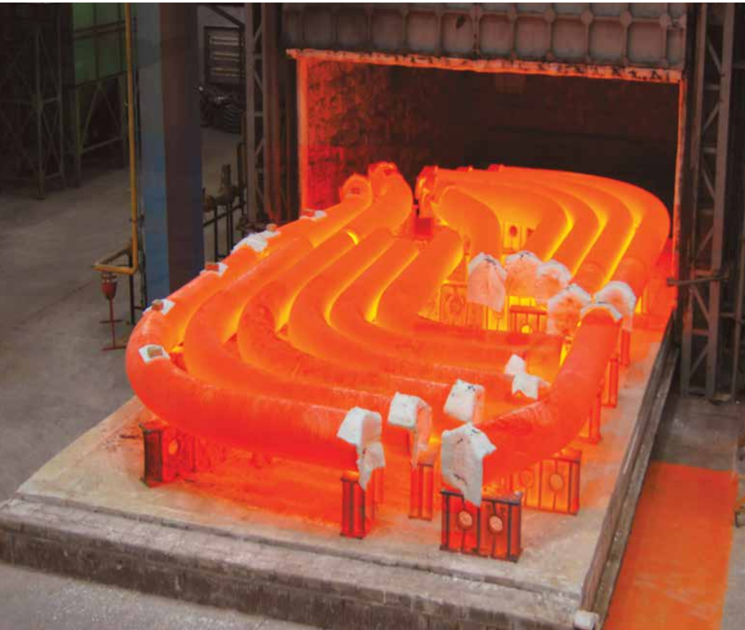
Critical Piping Spools undergoing heat treatment
