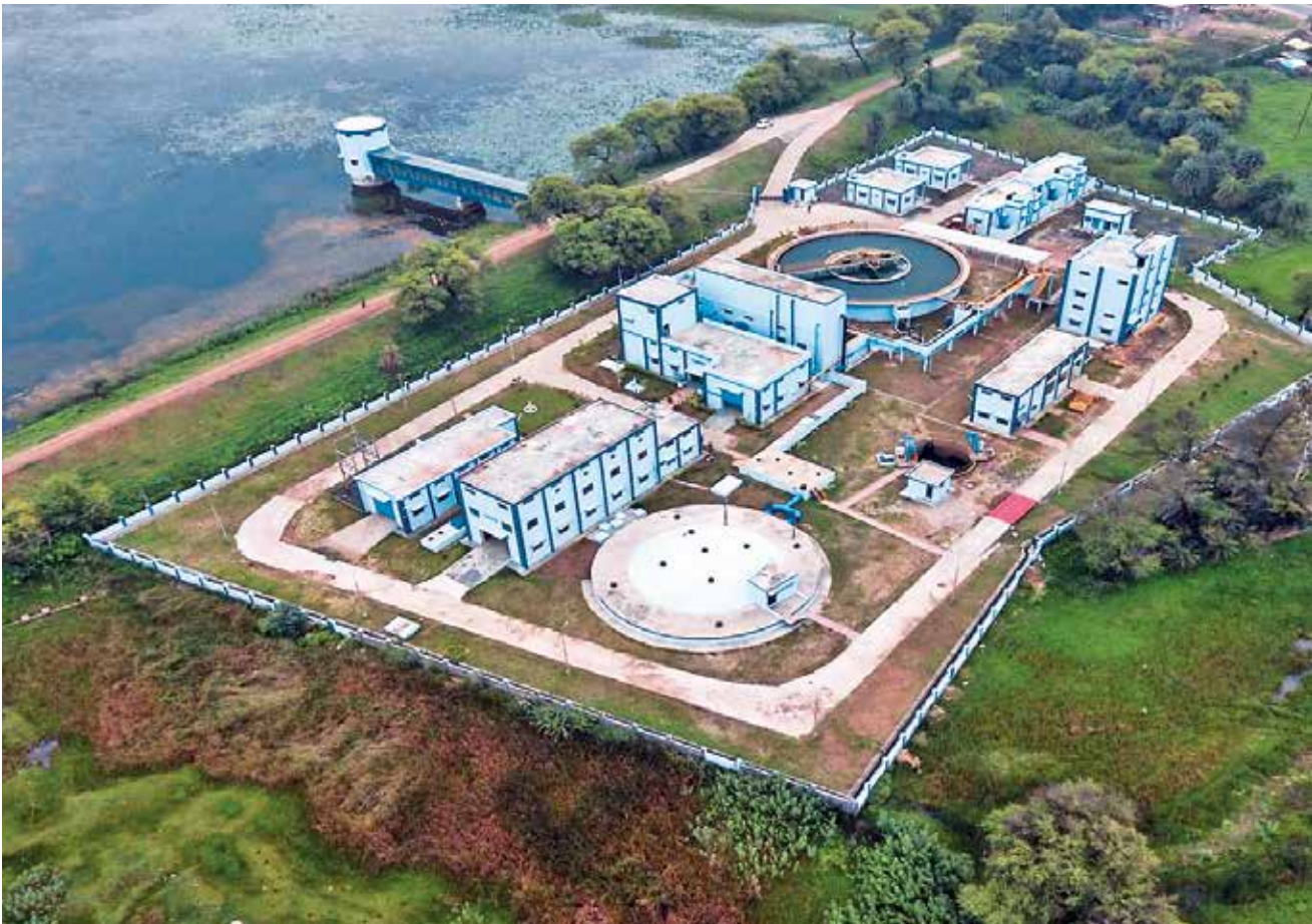
10.6 MLD Water Treatment Plant, Bagidora, Rajasthan
