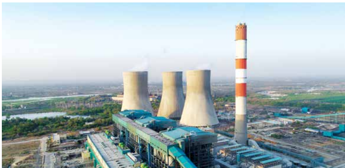
3x660 MW Koradi Thermal Power Plant, Maharashtra
