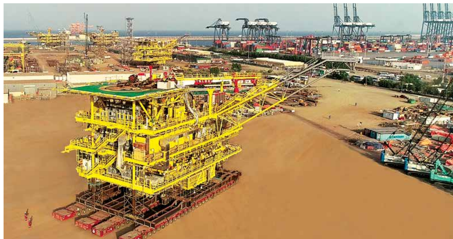
Six Gas Production Modules and two mega Tie-in Platforms (7000 MT each) for Hasbah II fabricated at LTHE's Oman Facility
