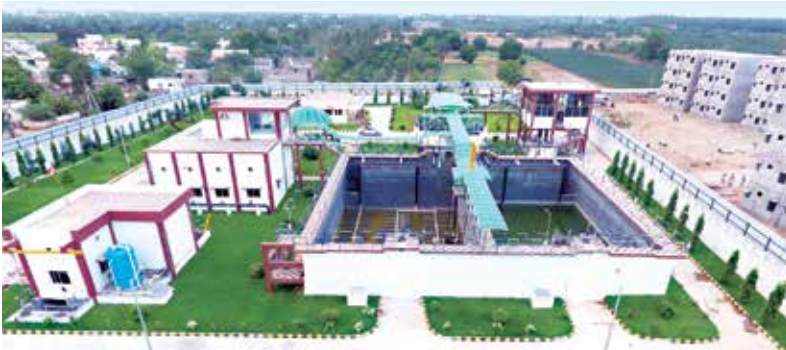
55 MLD Sewage Treatment Plant, Nellore, Andhra Pradesh
