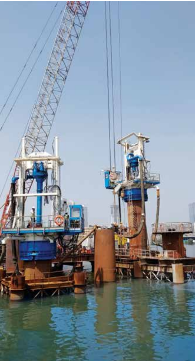
Reverse Circulation Drilling (RCD) rigs in operation at MTHL, Mumbai
