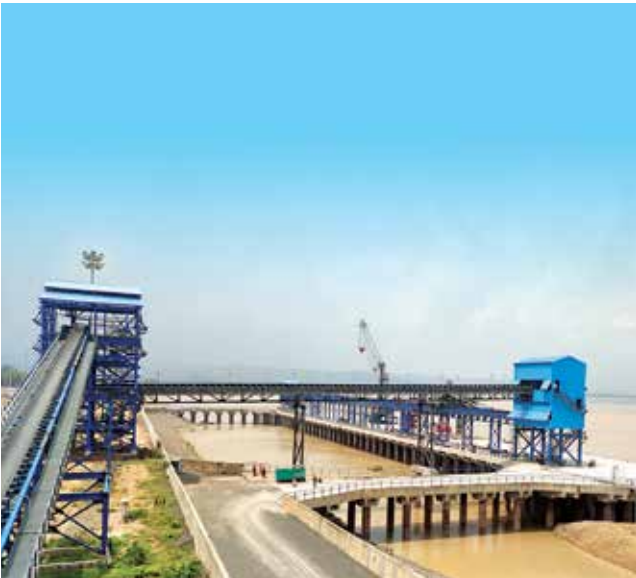
Multi-modal terminal at Sahibganj, Jharkhand
