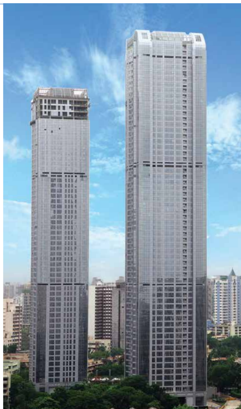
ICC Towers, Mumbai
