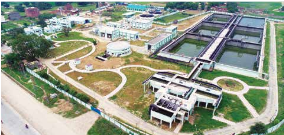
120 MLD Sewage Treatment Plant, Varanasi, Uttar Pradesh
