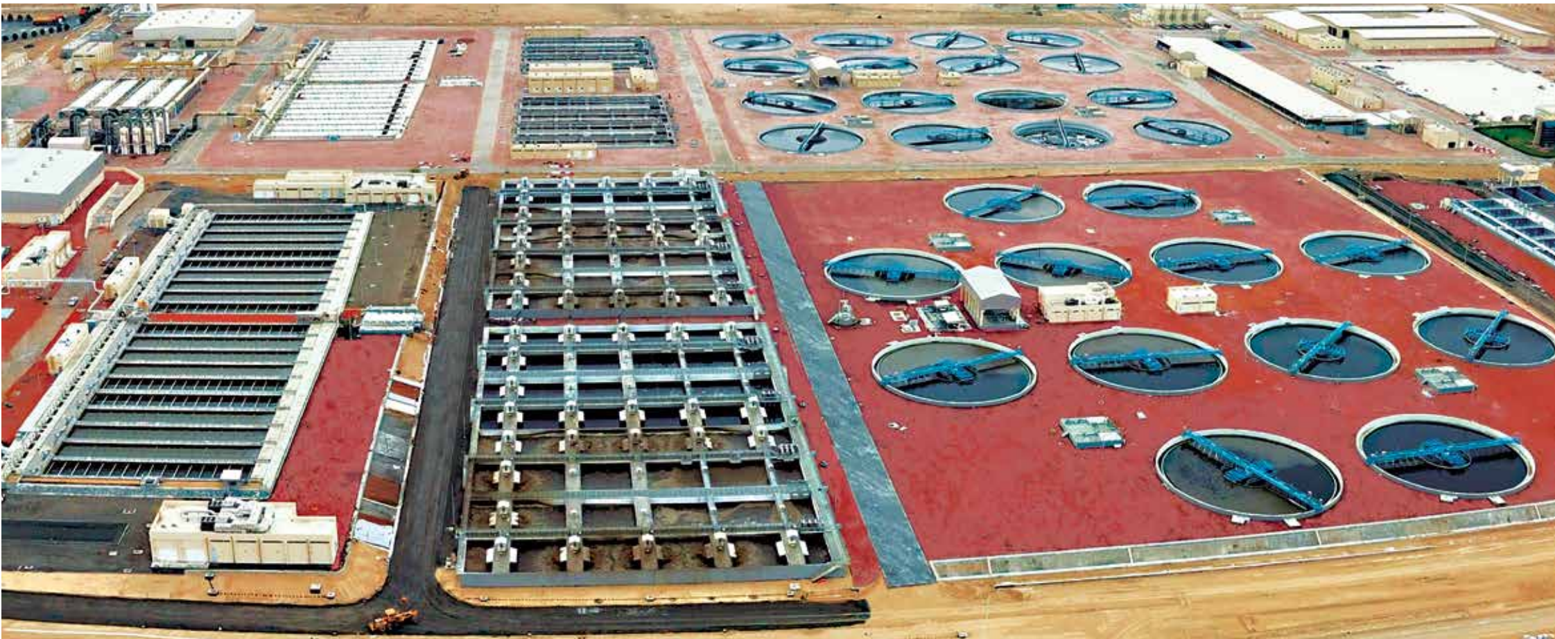
375 MLD Sewage Treatment Plant, Jebel Ali, UAE
