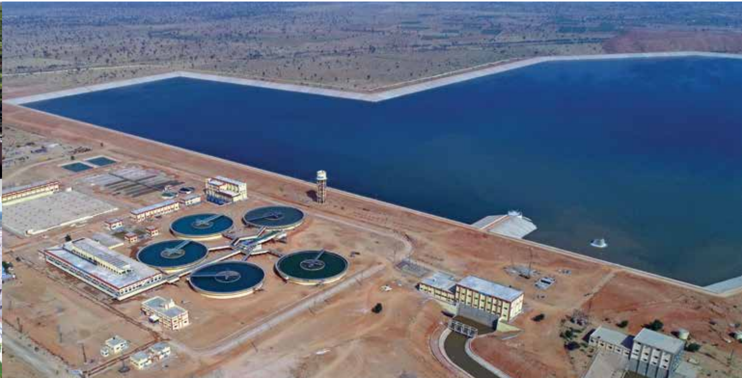
250 MLD Water Treatment Plant, Nagaur, Rajasthan
