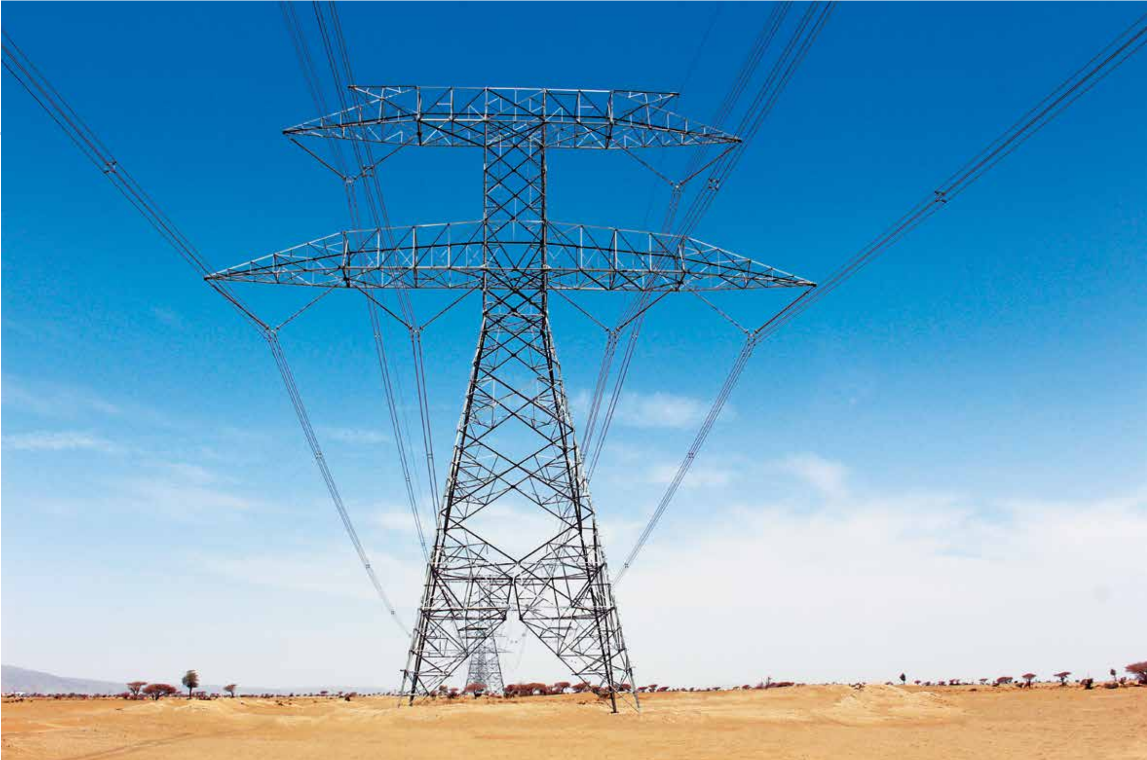
400 kV Ibri-Izki Transmission Line, Oman
