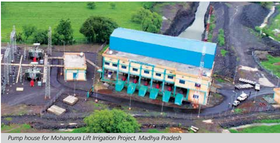
Pump house for Mohanpura Lift Irrigation Project, Madhya Pradesh
