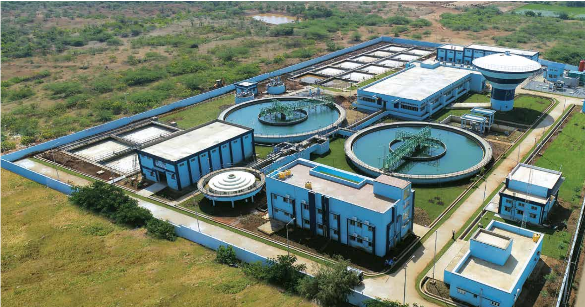
48 MLD Water Treatment Plant, Gadag, Karanataka
