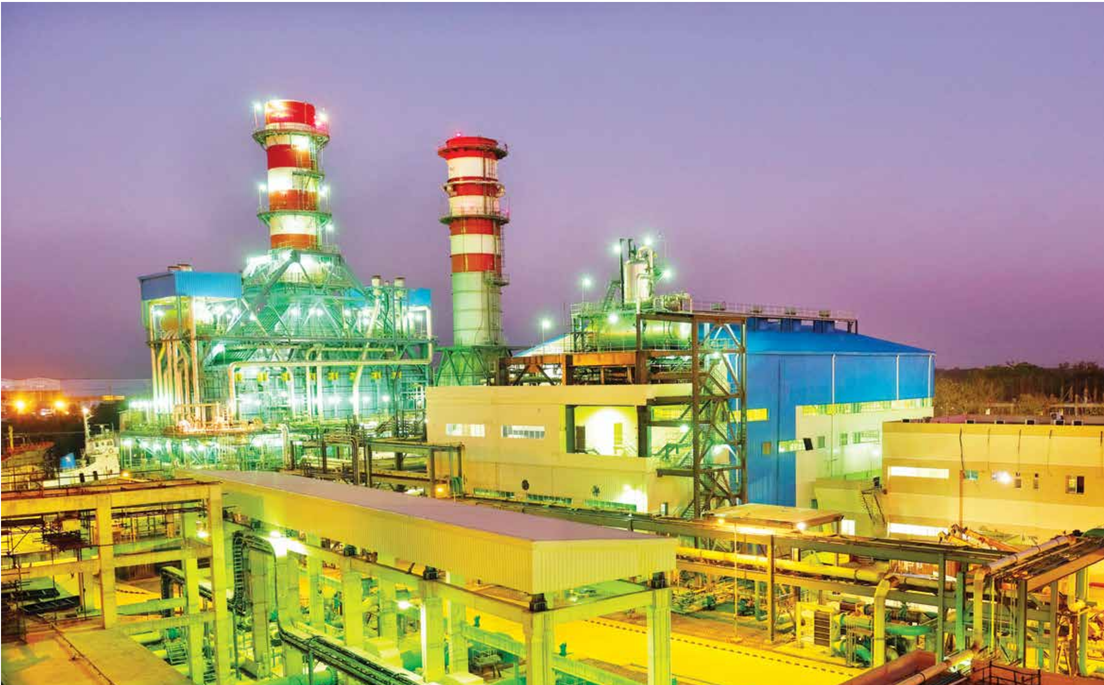
225 MW Sikalbaha Combined Cycle Power Plant, Bangladesh
