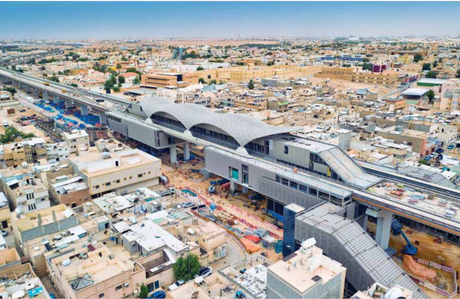
One of the stations of Riyadh Metro
