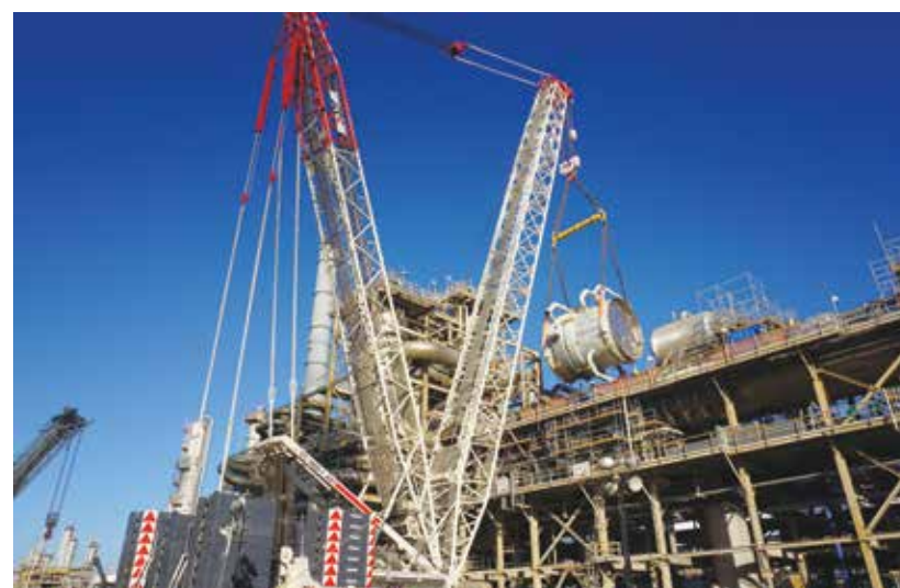
MRU - Critical Heat Exchanger Replacement at Kuwait
