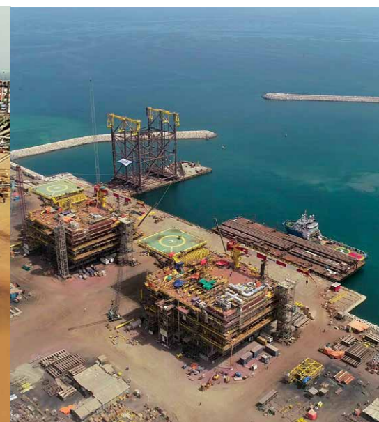
Two mega tie-in platforms (7000 MT each) for Saudi Aramco under fabrication at Oman Facility
