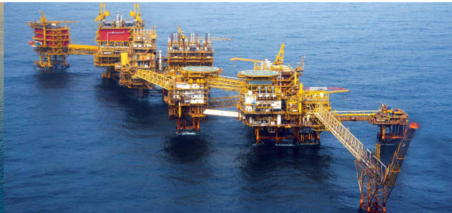
Bassein Development Project for ONGC. The scope included BCPA3 process platform, BLQ3 Living Quarters platform, BH wellhead platform, 12 km pipelines, bridges and modifications at BPA complex
