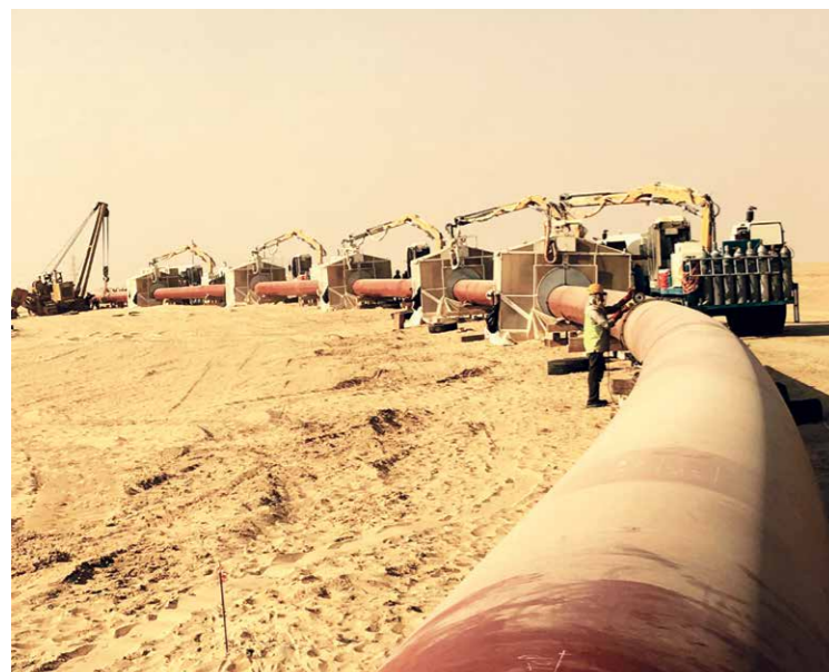
Laying of 125 km onshore pipeline from Land Fall Point to Fadhilli Gas Plant through Sabkha (Salt Pan) as part of onshore-offshore integrated Hasbah II Project, Saudi Aramco
