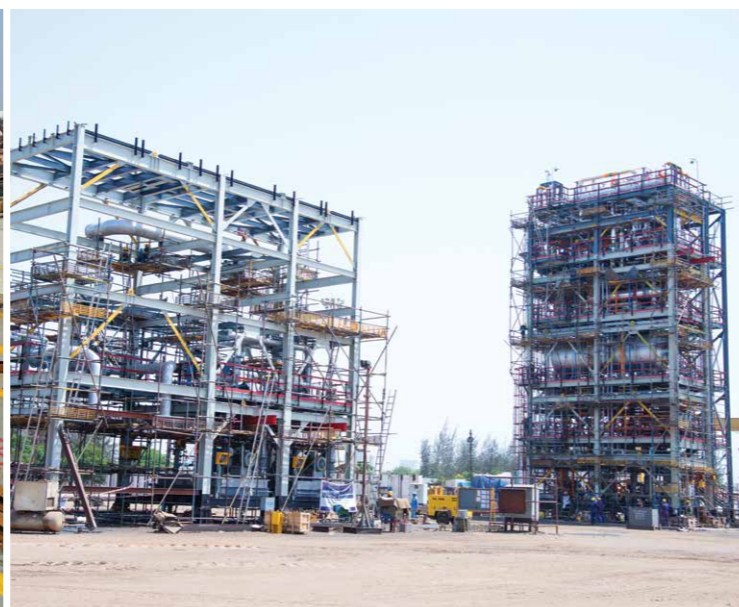
Modular Penex Unit and associated Off-Modules under fabrication for UOP / Bharat Oman Refineries Limited for Penex Revamp Project at Bina, India
