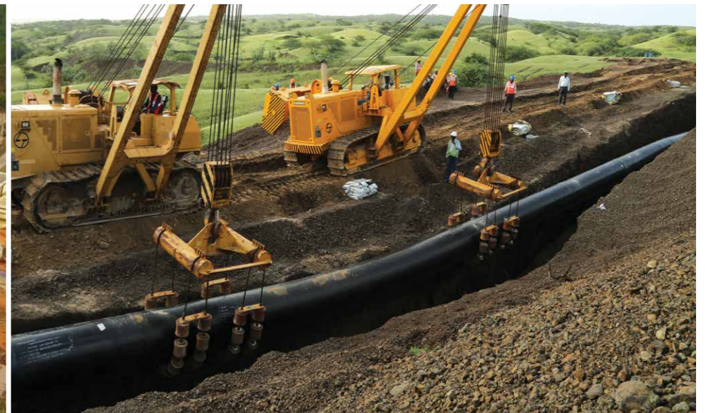
Laying of 36" x 67 km-long natural gas pipeline from Anjar to Mundra in Gujarat for Gujarat State Petronet Limited on EPC basis
