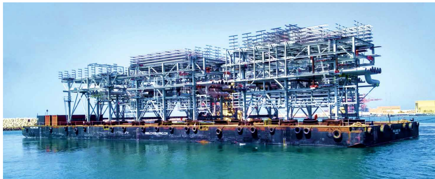
PAR modules for Al-Zour New Refinery Project of Kuwait Integrated Petroleum Industries Company (KIPIC). The scope includes 60 modules with a total weight of 7,500 MT
