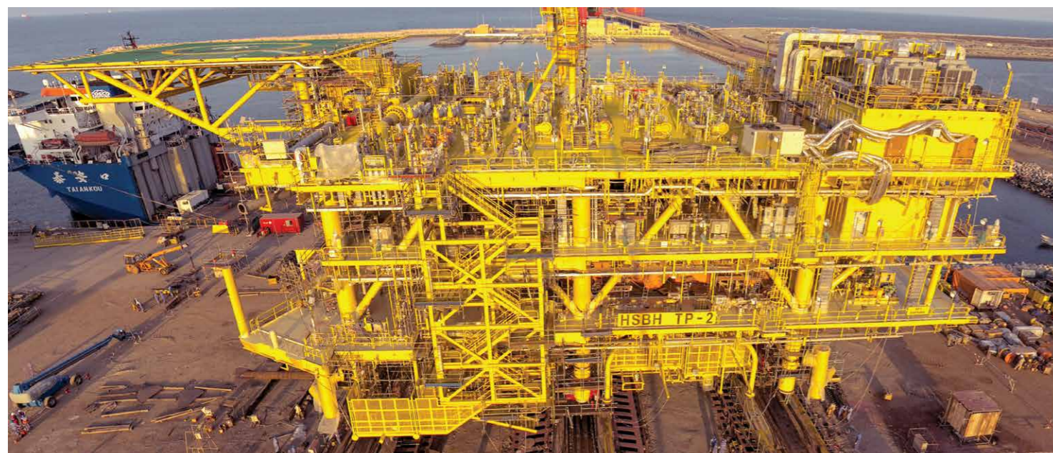
Loadout of Topside (7,000 MT) from Modular Fabrication Yard, Oman, for Saudi Aramco's Hasbah II Gas Increment Project
