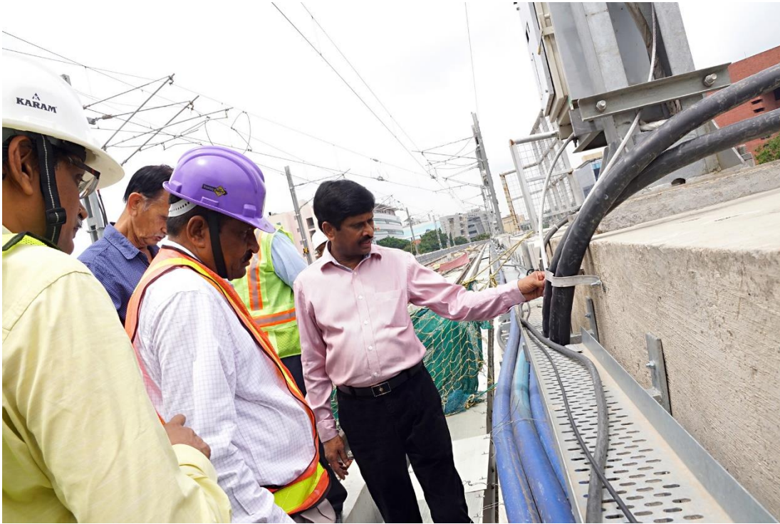
Mr. DVS Raju along with officials inspecting OHE works
