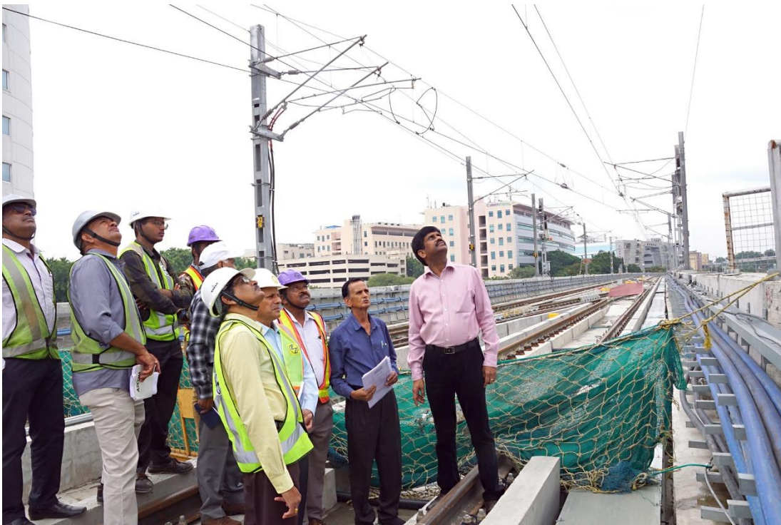
Mr. DVS Raju along with officials inspecting OHE at Raidurg
