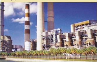
This plant located in Tampa Florida, consist of Units 1 and 2 – 460 MW each, Unit 3 – 470 MW and Unit 4 – 490 MW based on bituminous PRB. S&L's overall scope covered the detail design for retrofit SCRs on all four units at Big Bend. This included complete design and procurement of the SCR reactor and all ductwork, including duct internals. S&L was also responsible for all BOP design and procurement of all BOP equipment, including draft system modifications, foundations, steel, electrical, etc.
