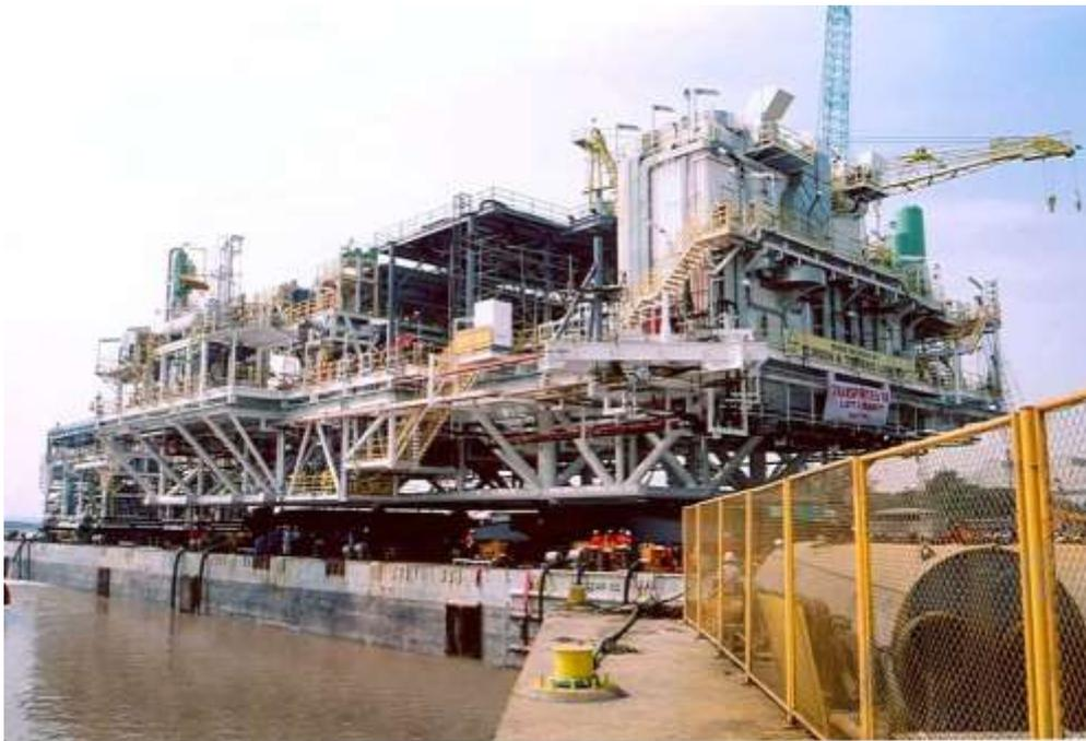
The 2400-tonne process platform built by L&T begins its 2500-km journey from L&T's Modular Fabrication Facility at Hazira, Surat to the El Bunduq oil fields of Abu Dhabi. The giant platform will be installed at site by January 16, 2006 – as part of the \$52.5 million Engineer-Procure-Construct contract secured by L&T.
