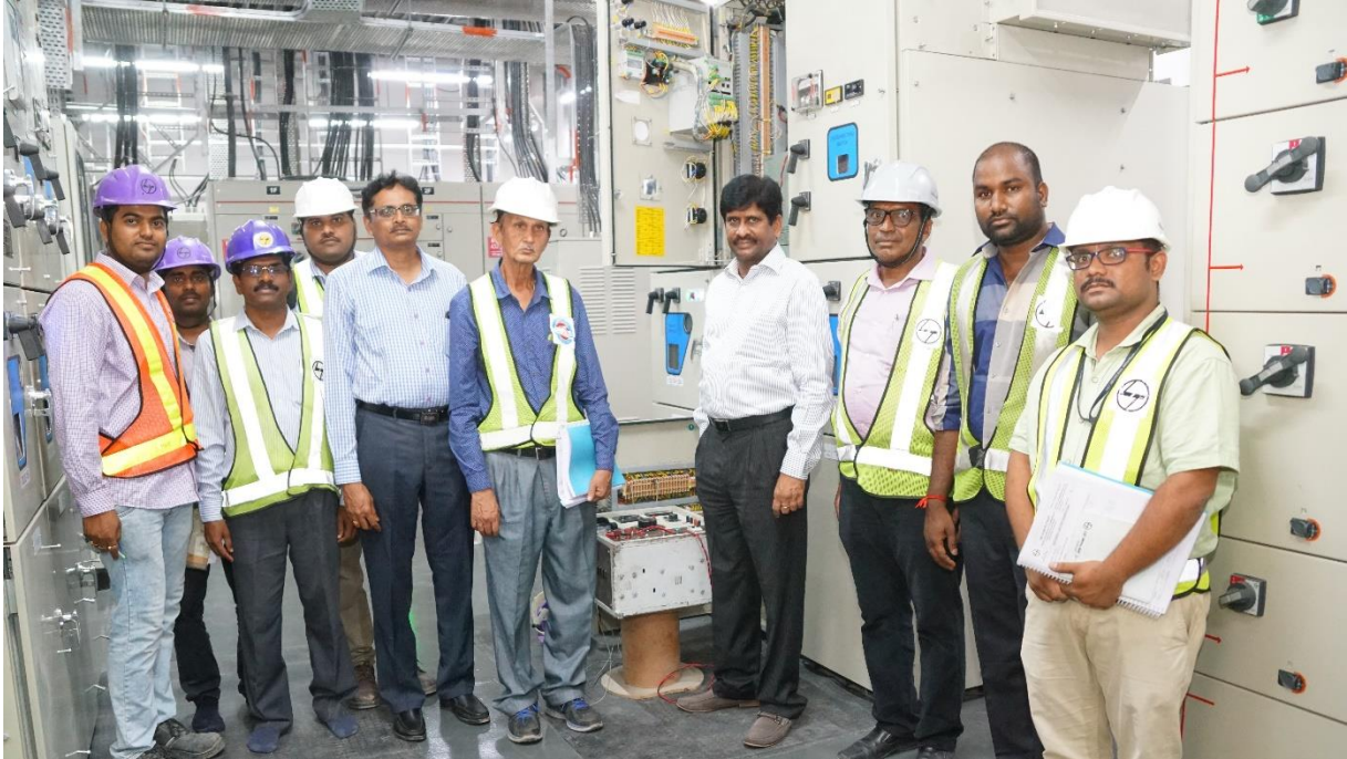
Mr. DVS Raju, CEIG, along with Mr. P. Srinivasa Murthy, Head - Electrical & MEP, LTMRL, Mr. H S Ananda, Dy. Chief Electrical Engineer, HMRL & AECOM.
