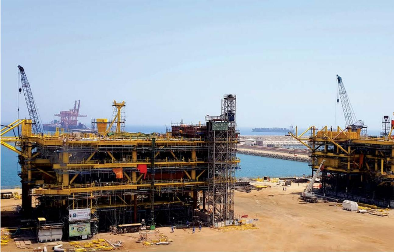
Two tie-in platforms, 7500 MT each, under fabrication at Modular Fabrication Yard, Oman, for Saudi Aramco's Hasbah II Gas Increment Project. The USD 1.6 billion project also includes six gas production deck modules, two six-legged jackets, pipelines, composite cables, umbilical and onshore valve stations.
