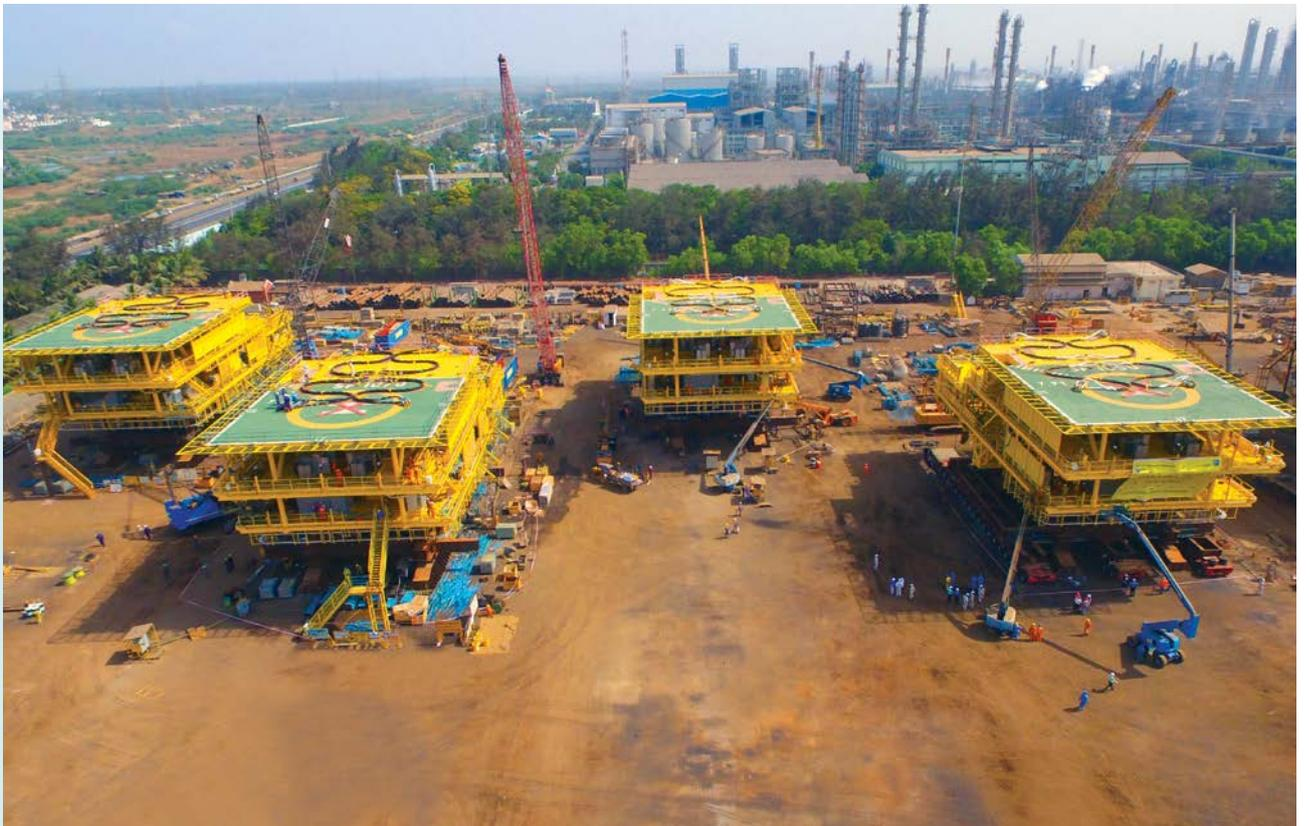
*Four Production Deck Modules for Saudi Aramco ready for despatch from Modular Fabrication Facility, Hazira to Safaniya Field, Saudi Arabia*
