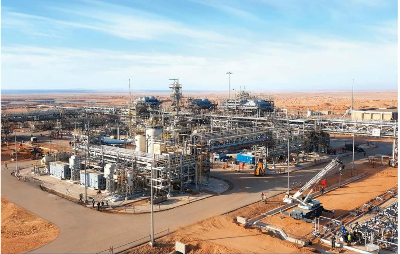
*Gas processing facilities for Saudi Aramco near Tabuk in Saudi Arabia, with a capacity to treat 75 MMSCFD of gas and 4500 BPD of condensate, and the laying of over 90 km of gas and condensate product pipelines*
