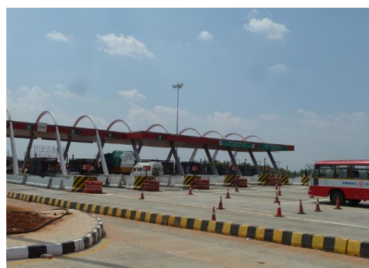
Figure 2.5: Km 169.5 Shantigramma Toll Plaza
