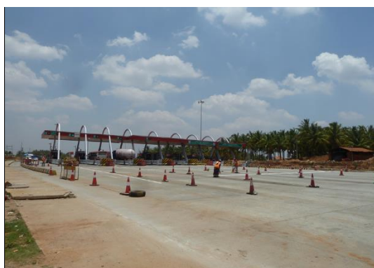
Figure 2.4: Km 119.1 Kadabahalli Toll Plaza
