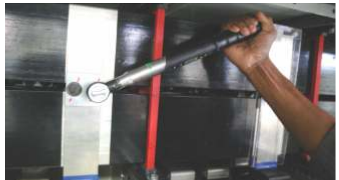
Figure 60 - Tightening of Busbar Joints
