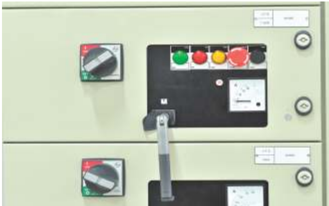
Figure 55 - Full width module in Test position
