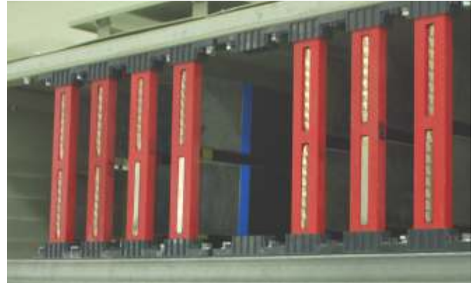
Figure 3 - Double Deck Arrangement of busbars
