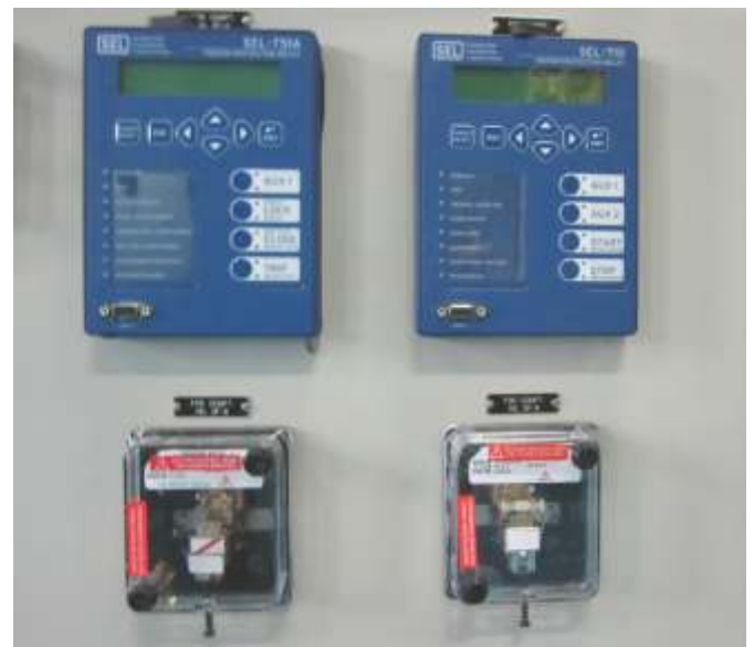
Figure 47 - Relay Mounting on Panel
