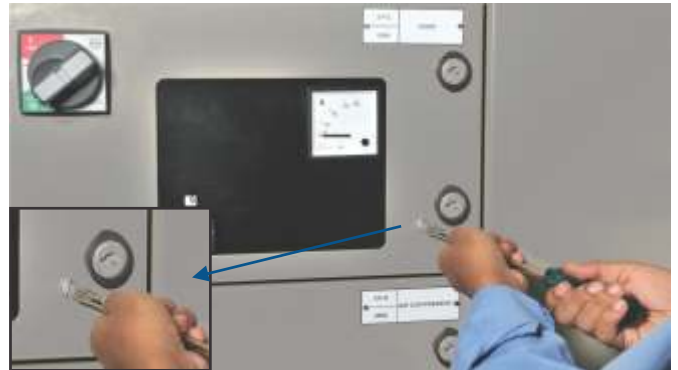
Figure 17 - Door defeat interlock
