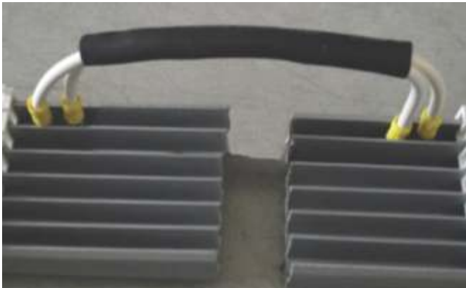
Figure 40 - Auxbus joining
