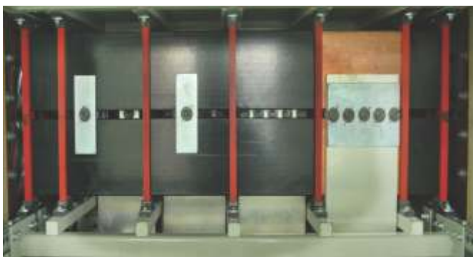
Figure 59 - Tightening of Busbar & Dropper Joint
