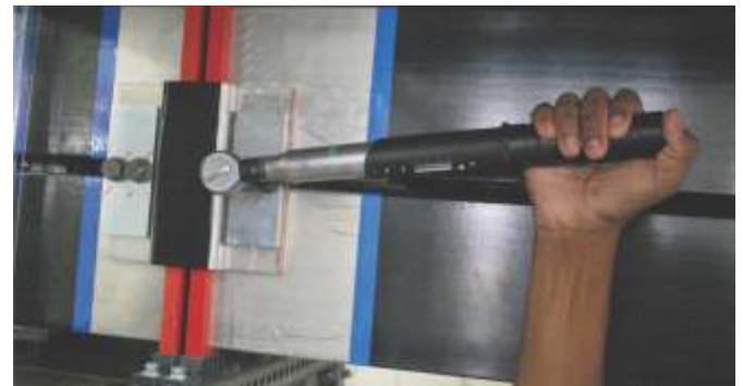
Figure 39 - Tightening of Busbar joints
