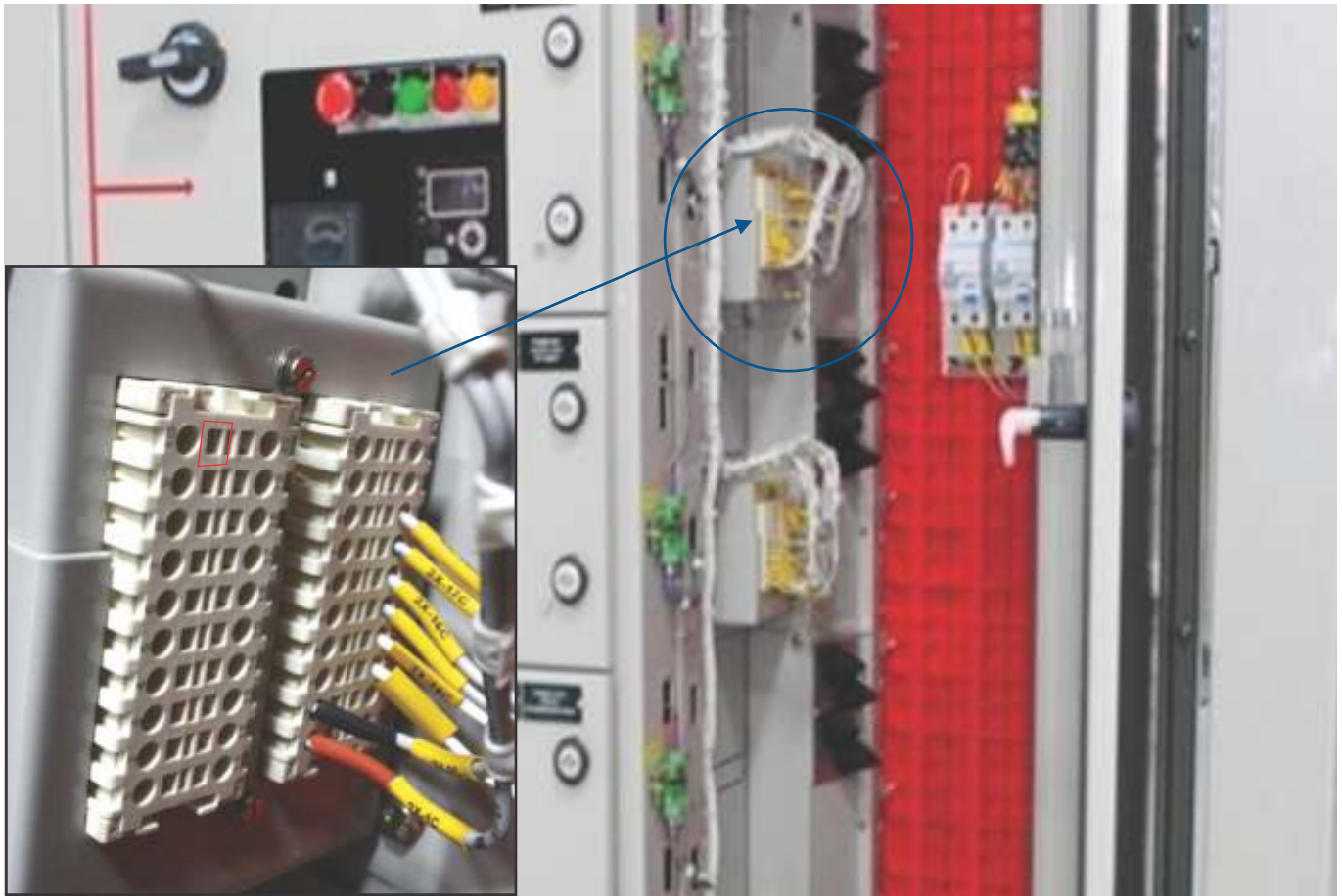
Figure 45 - Control Cable terminals
