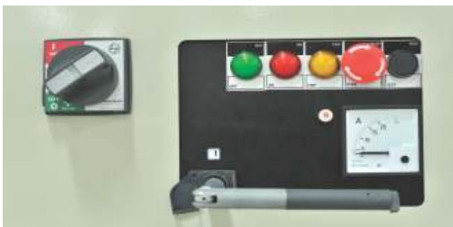
Figure 56 - Full width module in Isolated position
