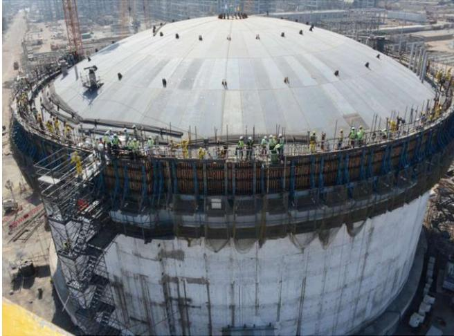
*Cryogenic Ethylene Tank – Dome Air Raising*
