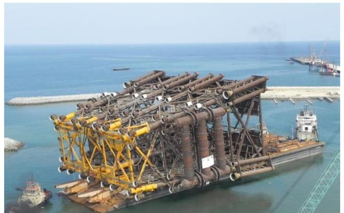
*Sail-away of jacket for Asia's largest process platform (13,500 MT, 8-legged launch-type with 23 pre-installed risers) from Modular Fabrication Facility at Sohar in Oman*
