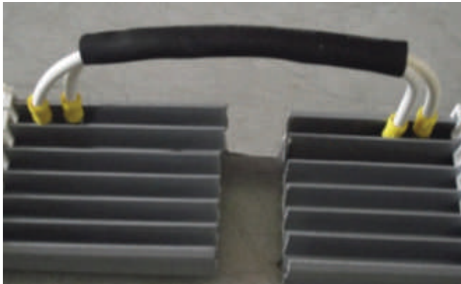
Figure 20 - Auxbus joining
