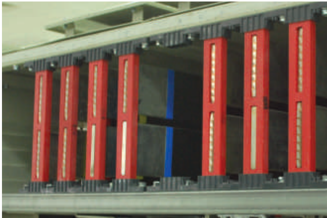
Figure 3 - Double Deck arrangement of busbars
