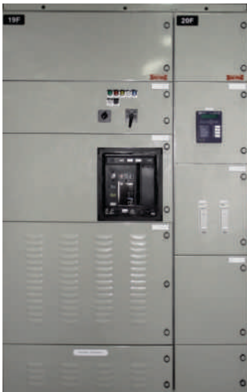
Figure 1 - Typical PCC panel
