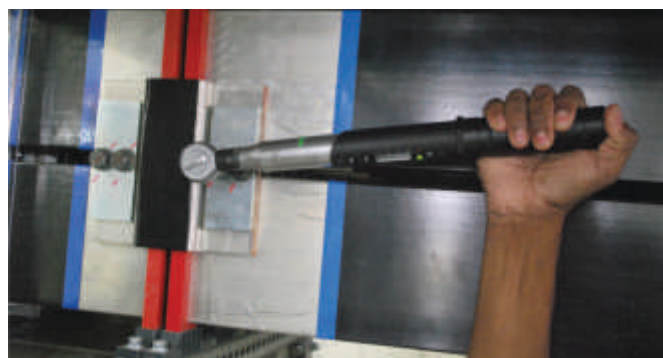
Figure 19 - Tightning of Busbar joints
