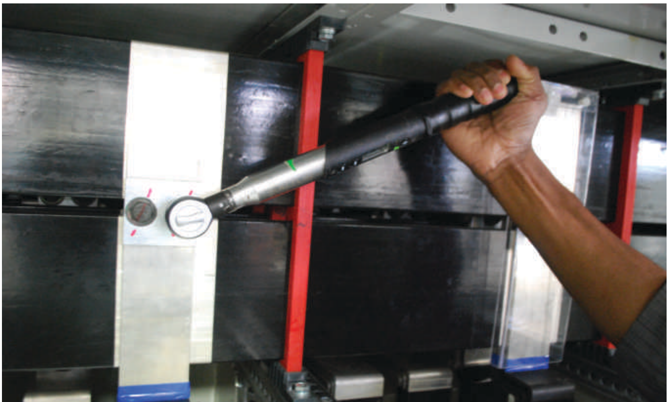
Figure 36 - Tightening of Busbar & Dropper Joint
