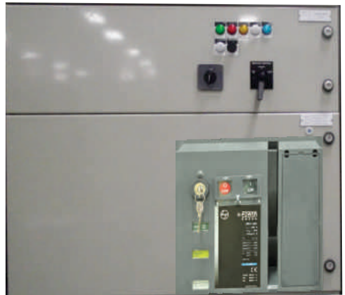
Figure 35 - Front facia of ACB
