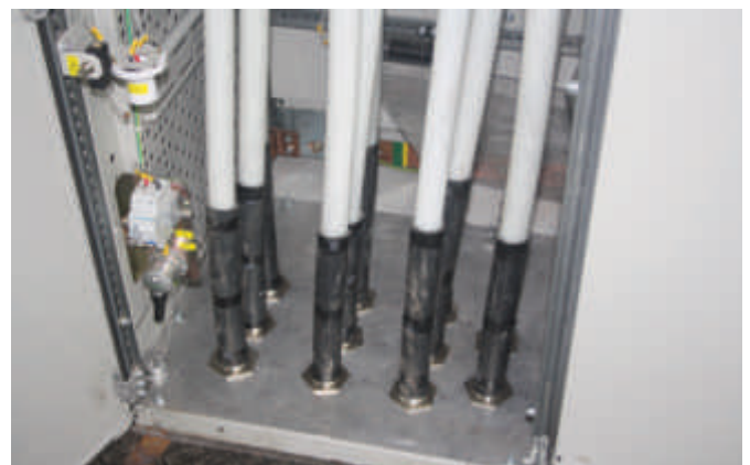
Figure 26 - Power cable terminals bottom cable entry
