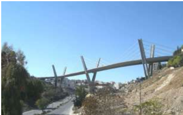
A view of the bridge.
