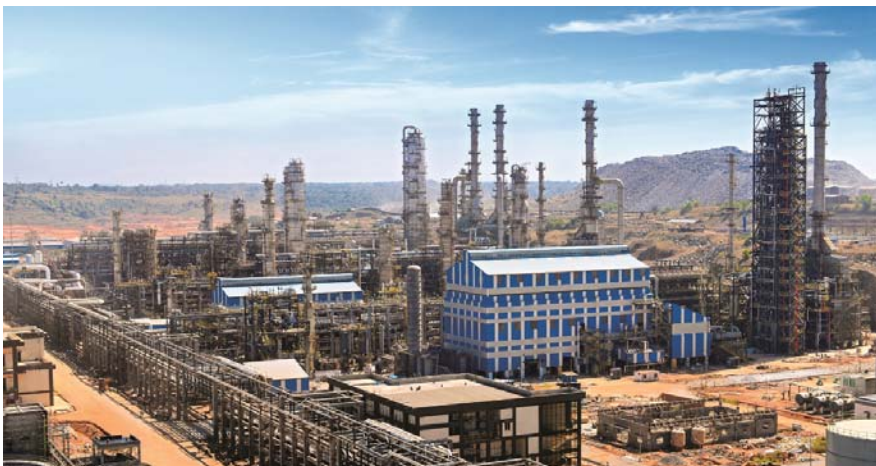
Mangalore Aromatic Complex built on LSTK basis
