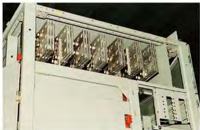
Interleaved arrangement of busbars
