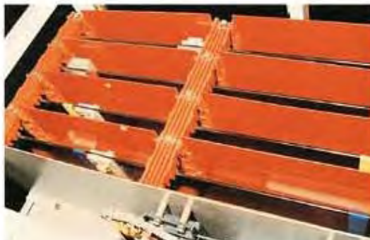
Interphase barriers for horizontal busbars
