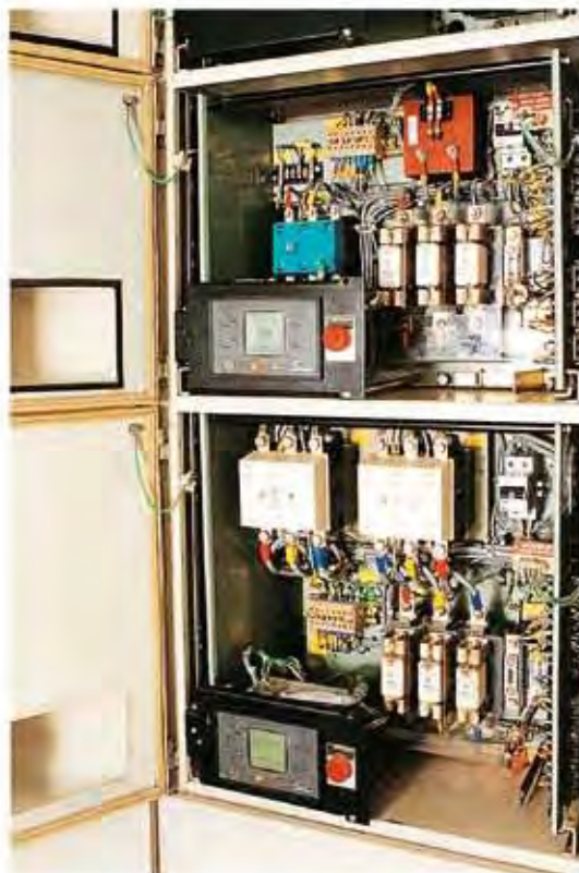
Starter feeder with intelligent relay
