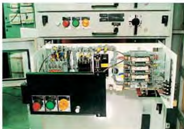
200mm module in maintenance position
