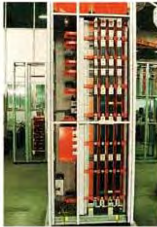
Completely sleeved busbars & droppers
