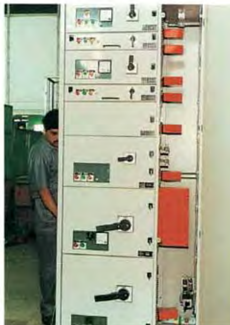
Completely shrouded power terminals offer operator safety
