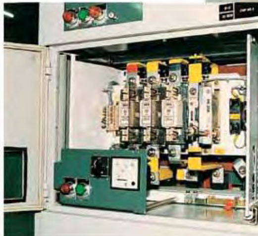
Module in Service position
