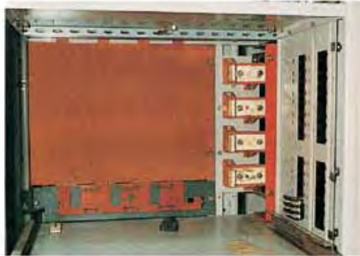
Safety shutter for incoming power contacts
