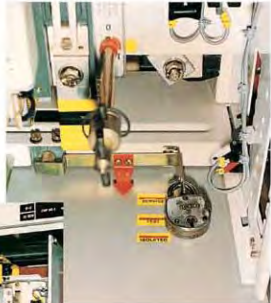
Module in Service position
