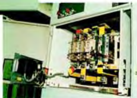
Control plate hinged for maintenance purpose
