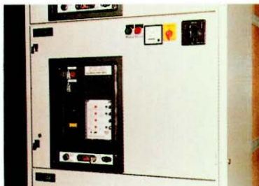
Compartment housing ACB with microprocessor based release.
