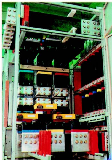
Interleaved link work for buscoupler
