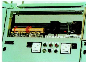
Auxiliary busbar arrangement and interpanel wire terminations.
