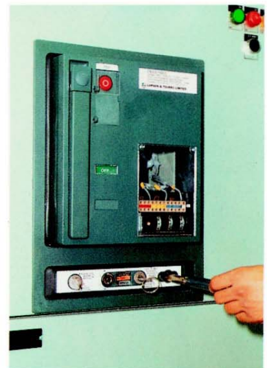
Storage slot for racking handle.
