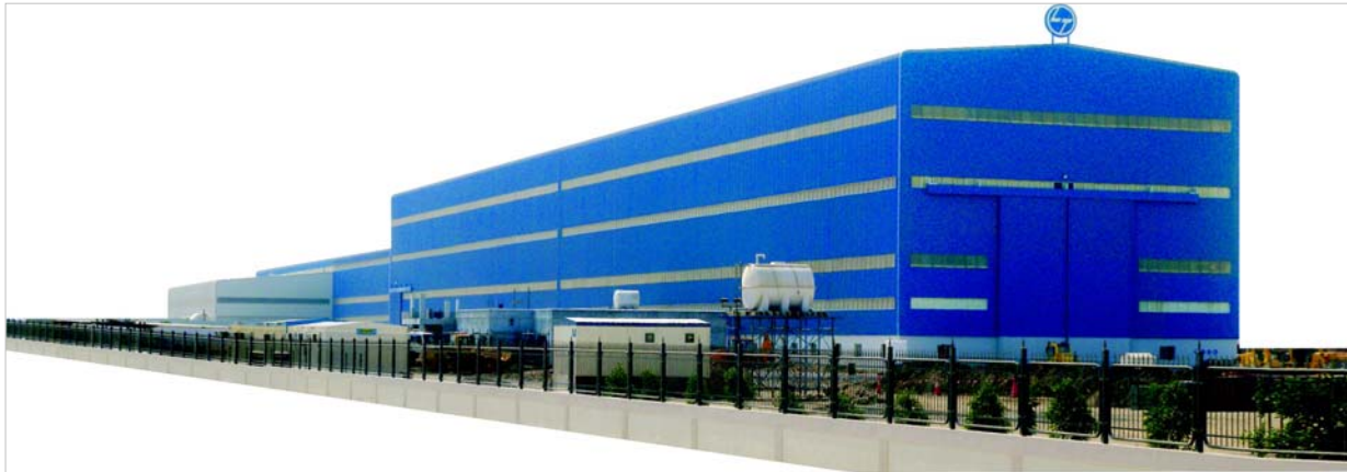
The Sohar heavy engineering facility.
