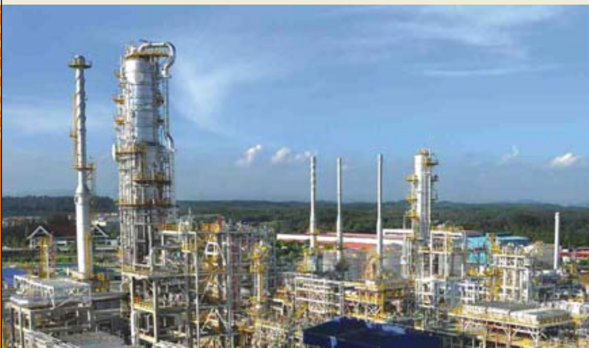
Stacks at Melaka Refinery, Malaysia
