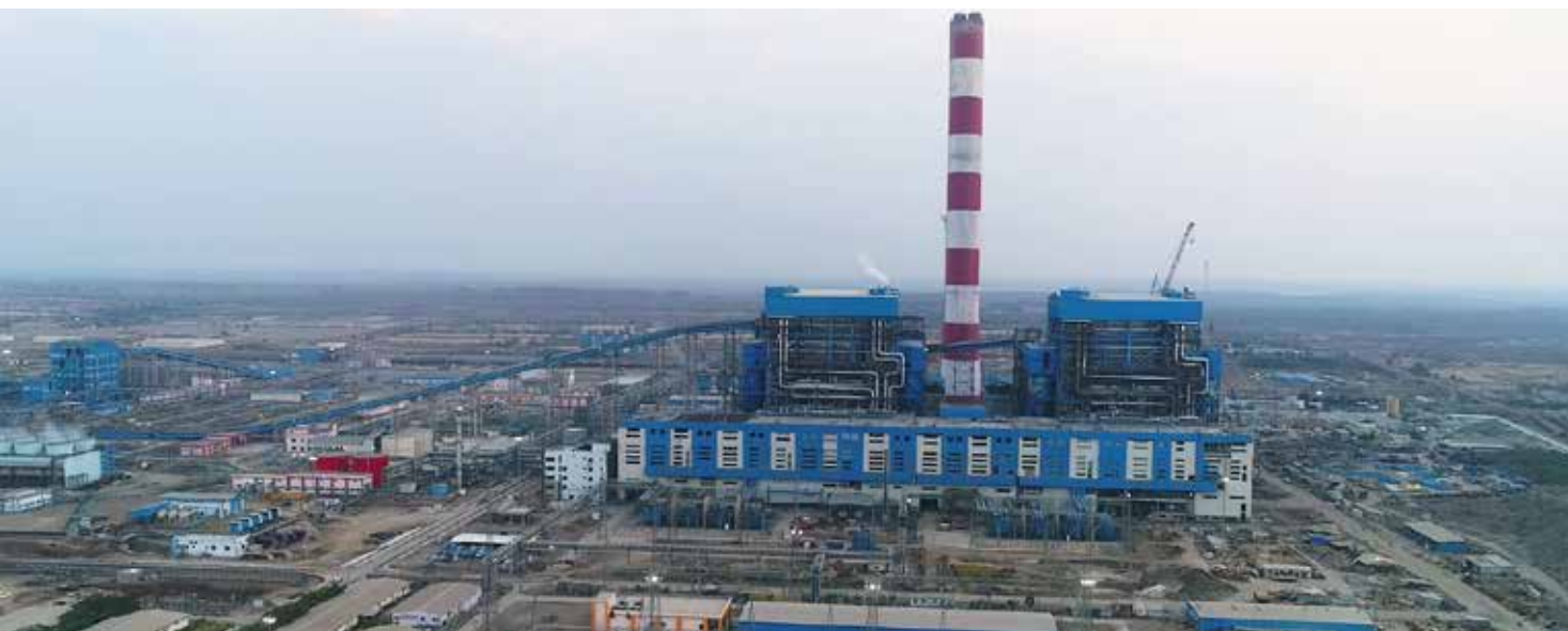
2x660 MW Khargone Thermal Power Plant, Madhya Pradesh, India
