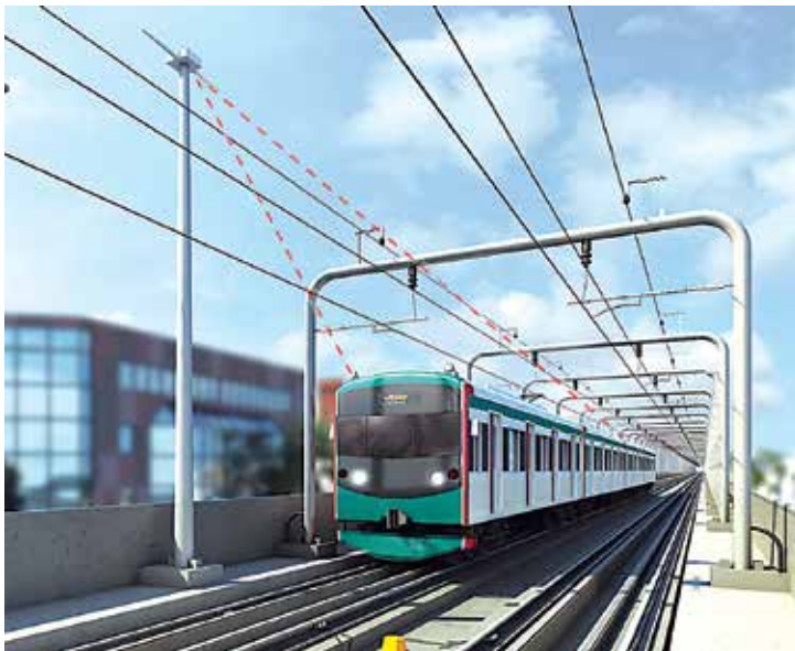
E&AM System Works, Dhaka Metro
