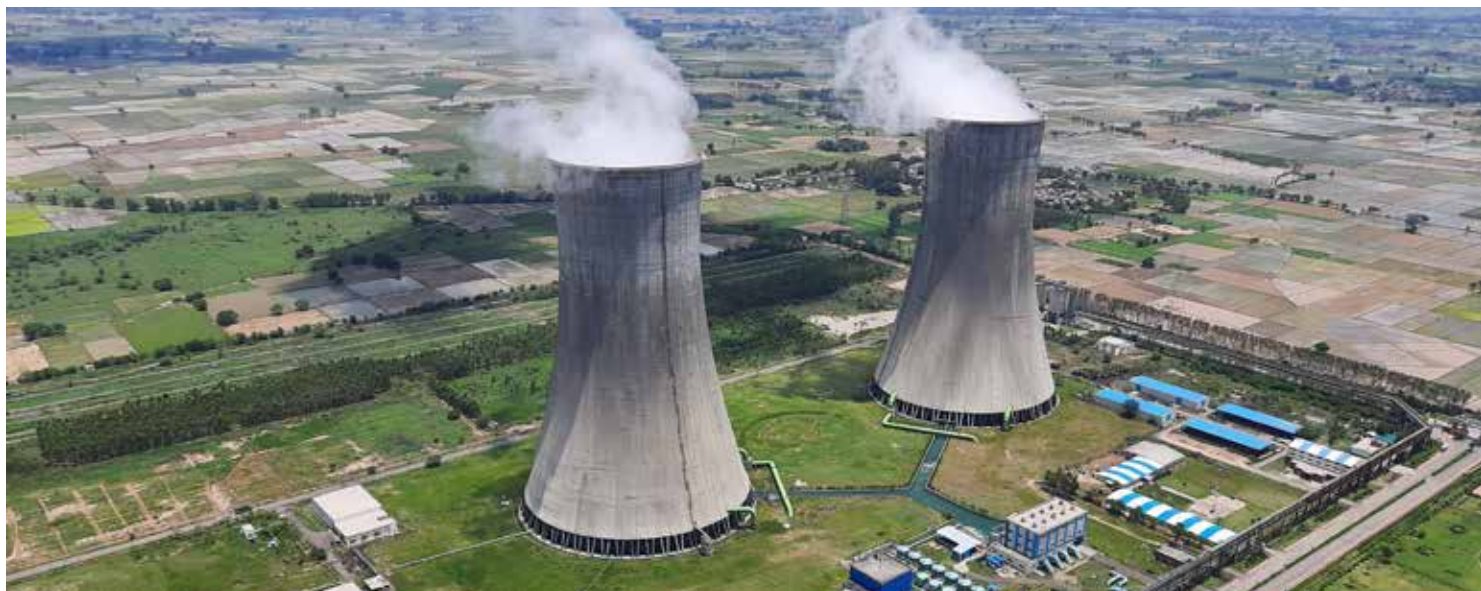
Aerial view of cooling towers, Rajpura Thermal Power Plant
