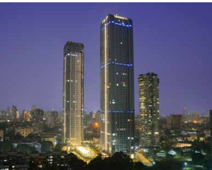
ICC Towers, Mumbai
