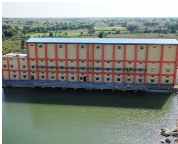
Pump house for Nandawadagi Lift Irrigation Scheme, Karnataka
