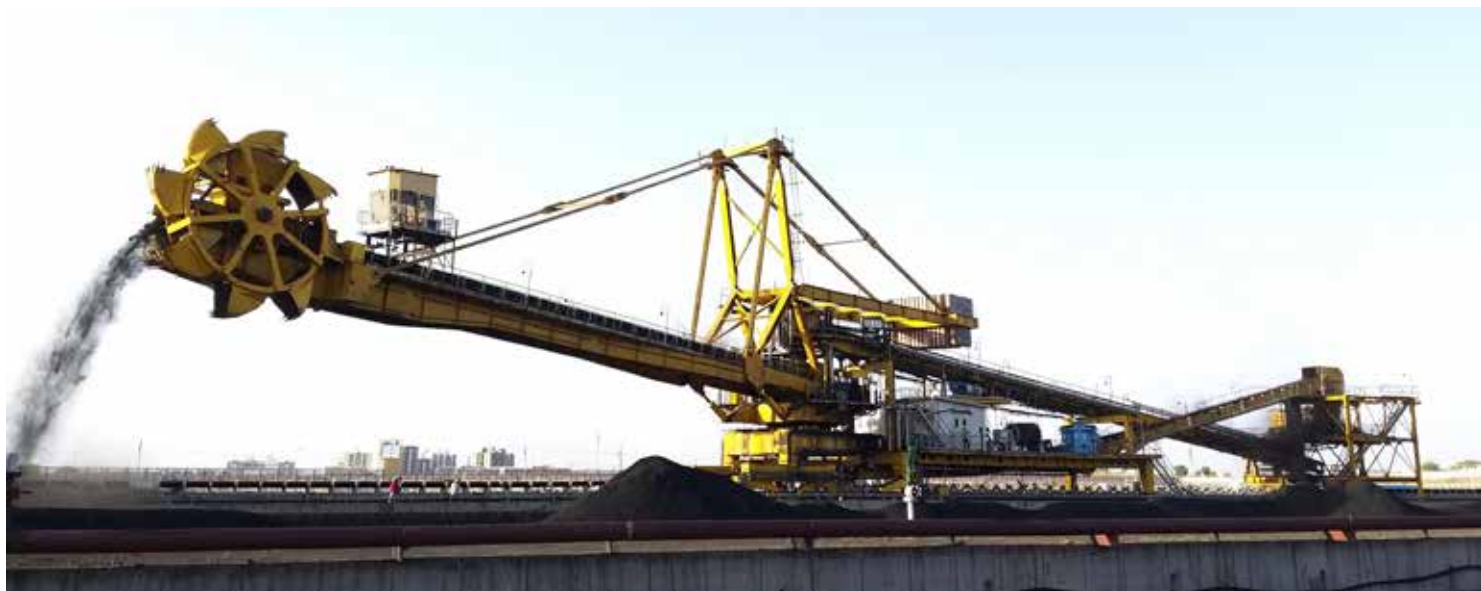
7C Stacker-cum-Reclaimer installed at Khargone
