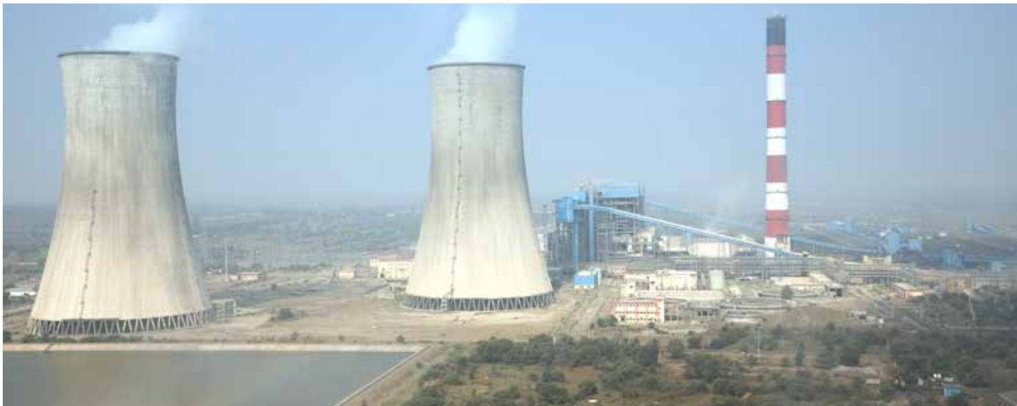
2x660 MW Chhabra Thermal Power Plant, Rajasthan, India
