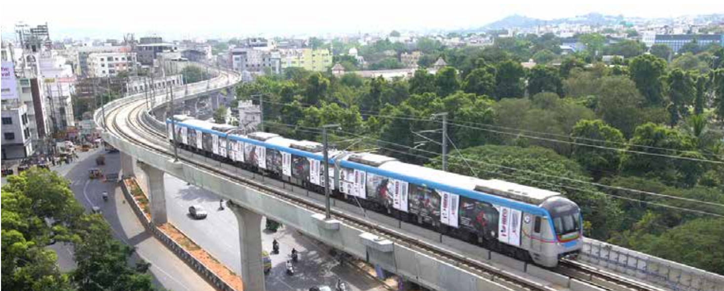
Hyderabad Metro Rail on the Viaduct
