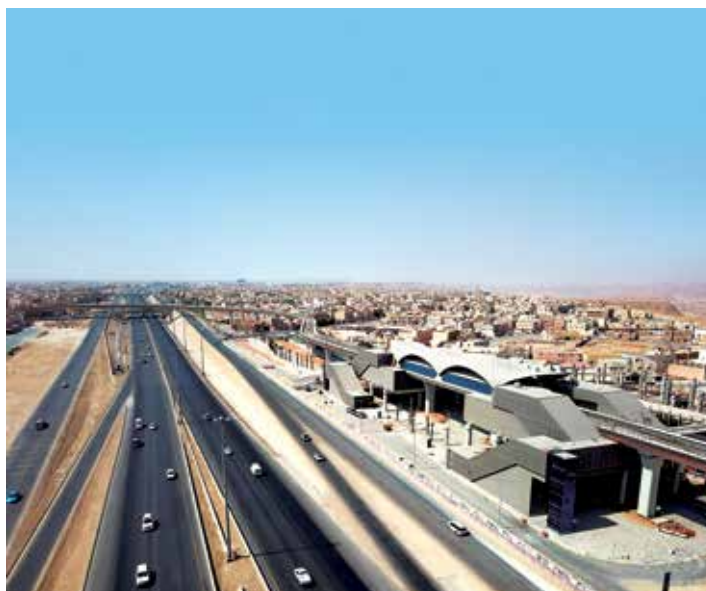
Riyadh Metro Line 3, Kingdom of Saudi Arabia
