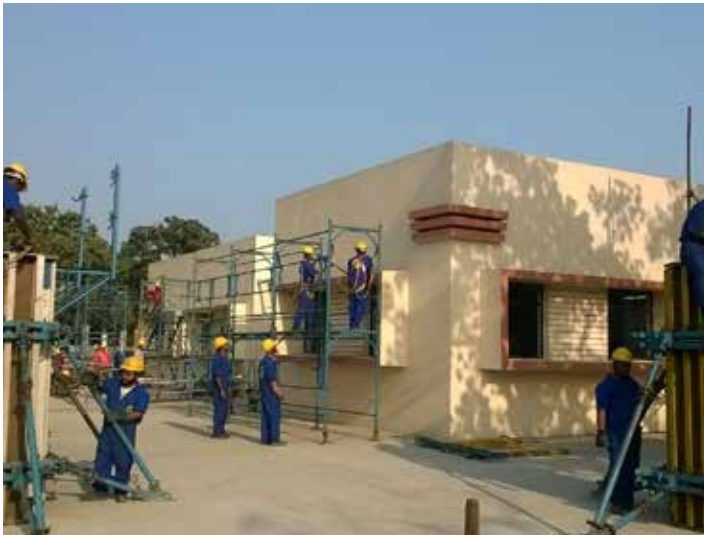
Scaffolding and formwork training at L&T's Construction Skills Training Institute (CSTI)
