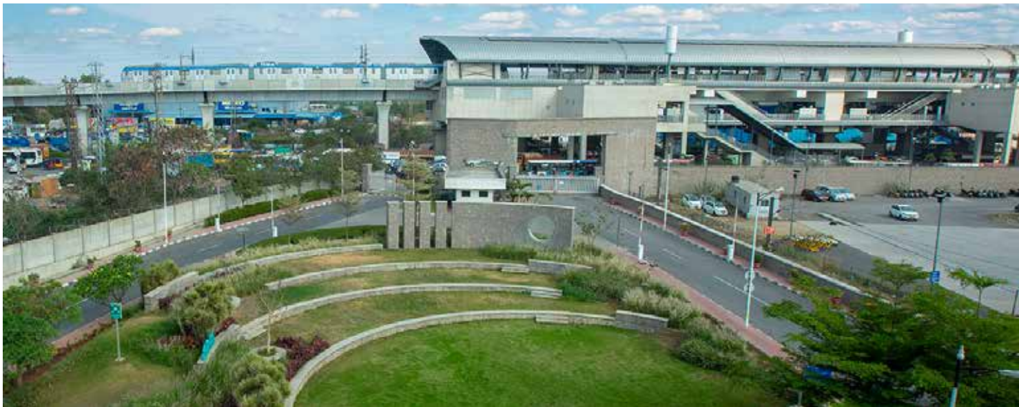
Hyderabad Metro Rail Uppal Depot and Nagole Station
