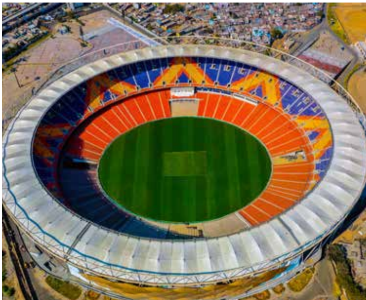
Motera Cricket Stadium, Gujarat
