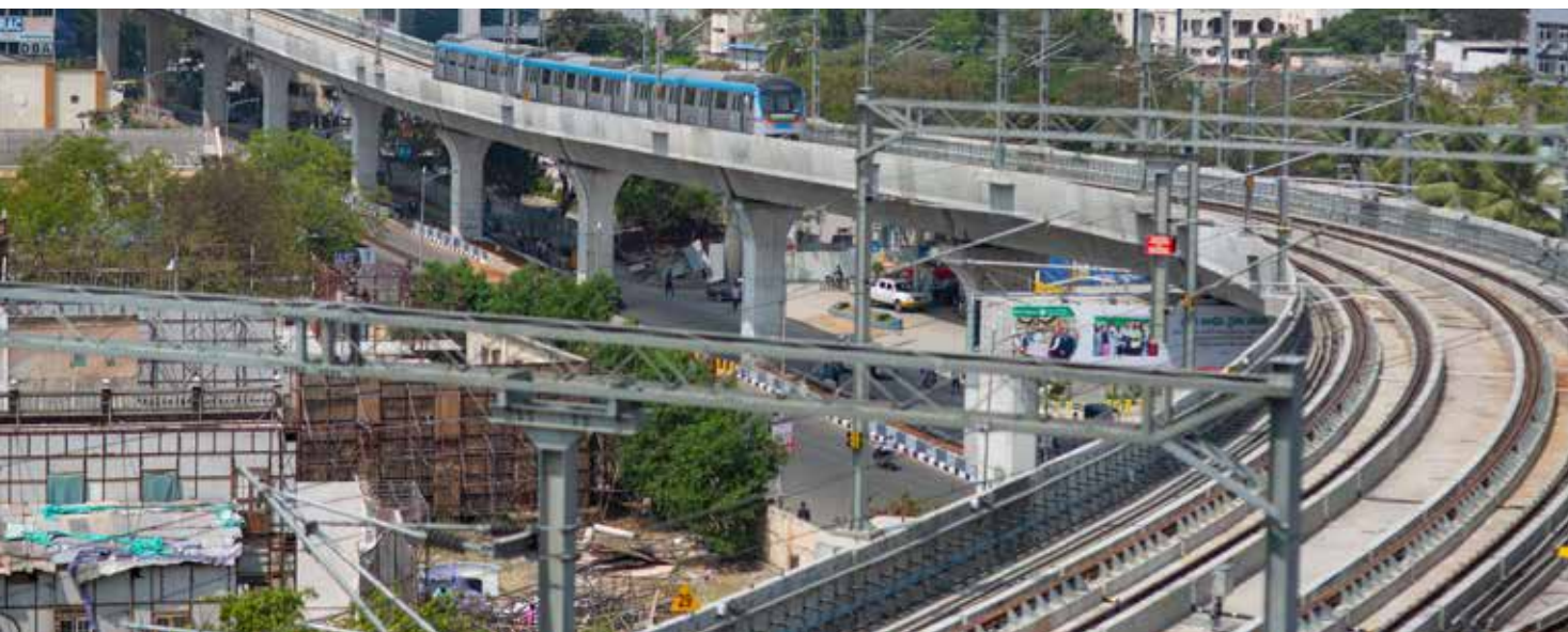
Sharp bend of the Viaduct
