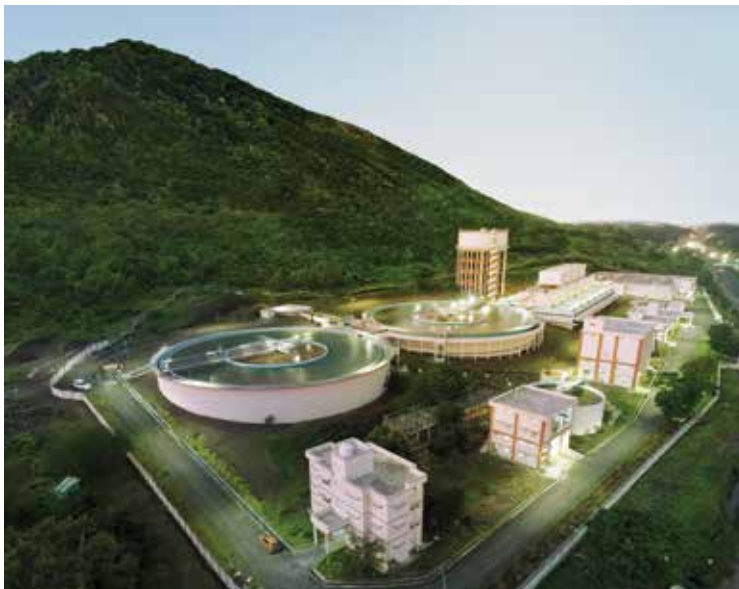
137 MLD Water Treatment Plant, Nashik, Maharashtra
