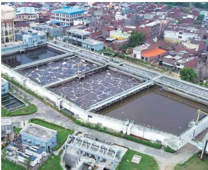
Moradabad Sewerage Treatment Plant, Uttar Pradesh
