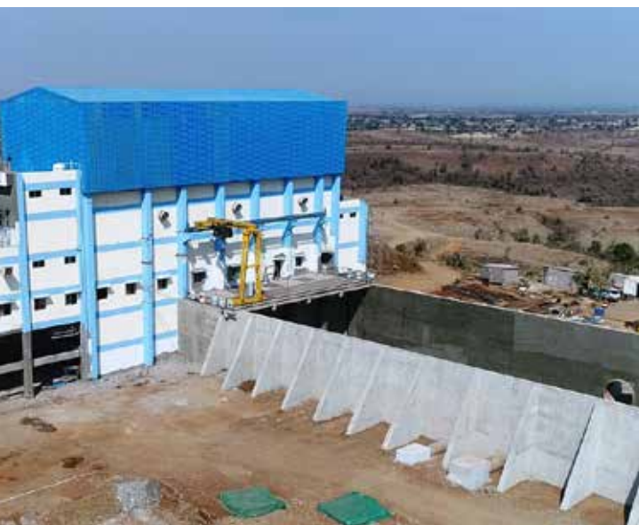
Pump house for Chhaigaonmakhan Lift Irrigation Scheme, Madhya Pradesh
