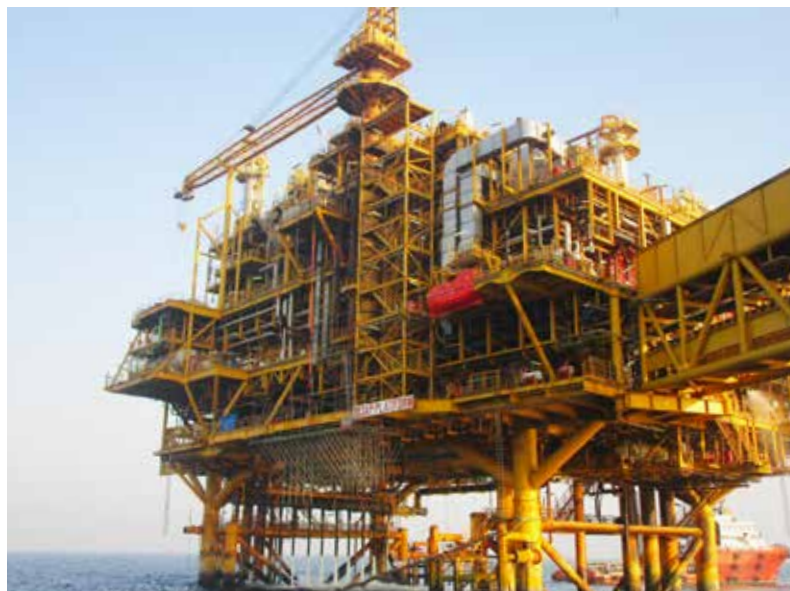
Bassein Development 3 Well Platform & Pipeline Project for ONGC
