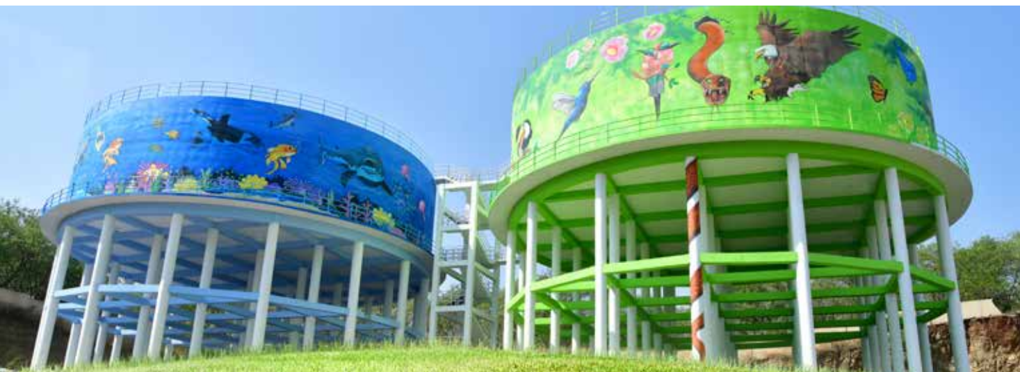
Elevated Storage Reservoirs at Pune, Maharashtra
