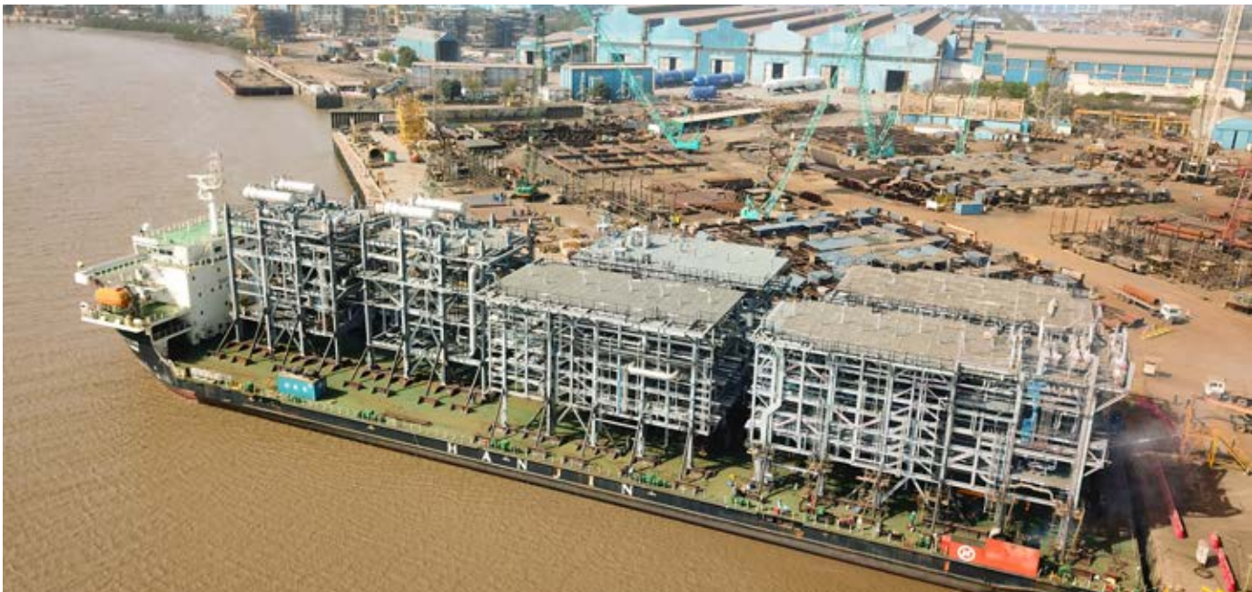
Onshore Process & Piperack Modules being loaded out from MFF Hazira for a Refinery in Thailand
