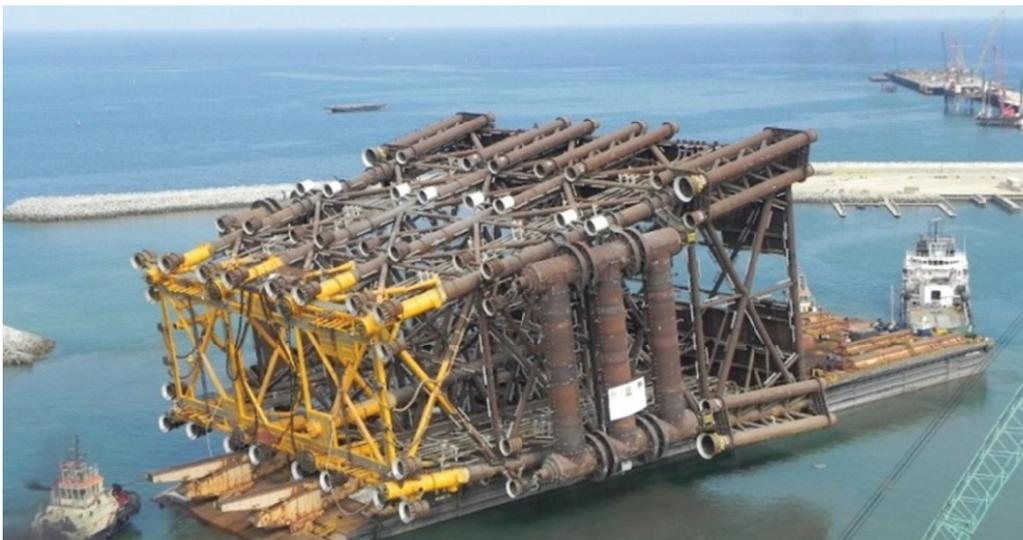
*Sail-away of jacket for Asia's largest process platform (13,500 MT, 8-legged launch-type with 23 pre-installed risers) from Modular Fabrication Facility at Sohar in Oman*
