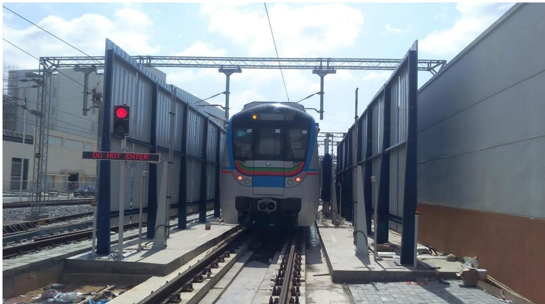
**Fig:-7 - Automatic Train Wash Plant**
