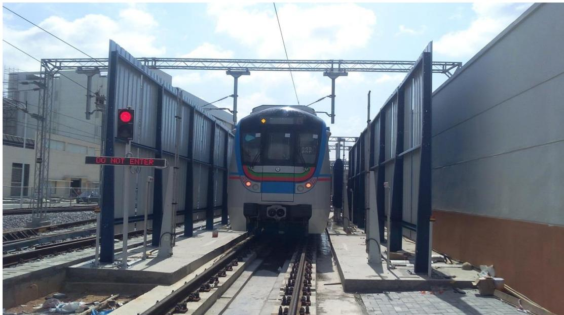
**Fig:-7 - Automatic Train Wash Plant**
