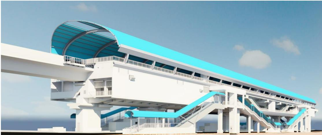
Stations being a window to Hyderabad Metro service are designed to integrate with the urban fabric of the city with minimum visual intrusion into the urban landscape. Typically a station is located above the road and consists of four levels, namely, Street, Concourse, Platform and Roof.
