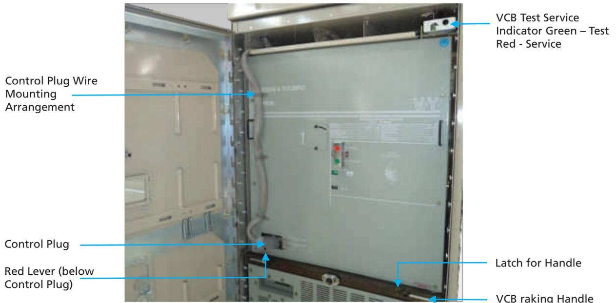
Figure 5.5 - Control Plug Arrangement
